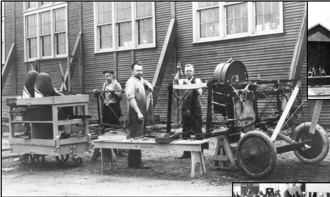
Above: Rebuilding an airplane fuselage at Fairfield Air Intermediate Depot, 1925. Employee in center is identified as the foreman, Mr. Erwin F. Boger.
