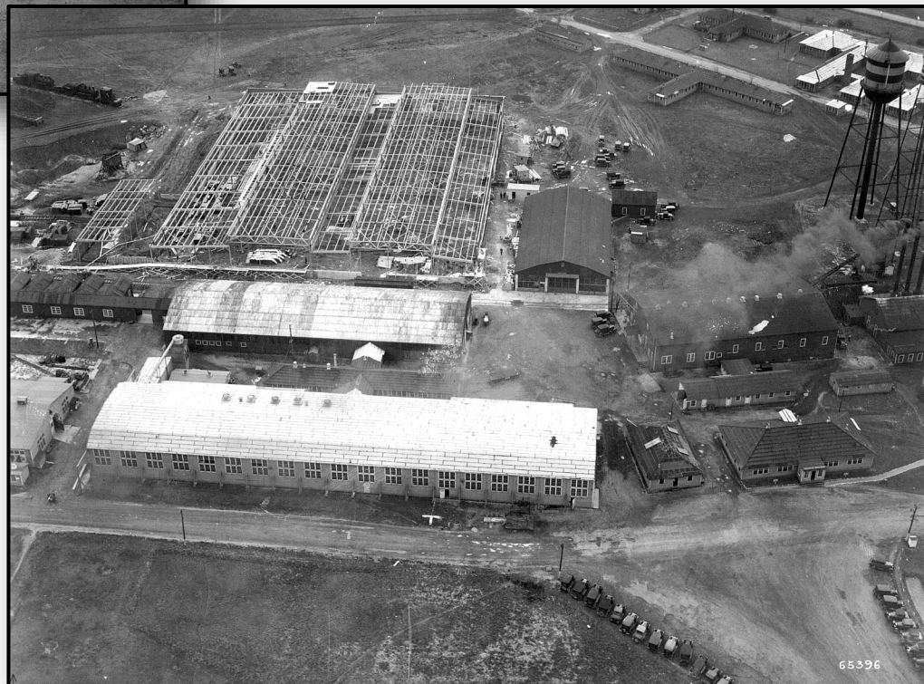
Right: Framework of Building 13, engineering department, being erected at Depot in early 1930. In later years the open space around this building was utilized with a heavy concentration of buildings and roadway of the engineering department. Not the absence of paved roads on the post and the smoke nuisance created by "little Pittsburgh," the main boiler plant.
