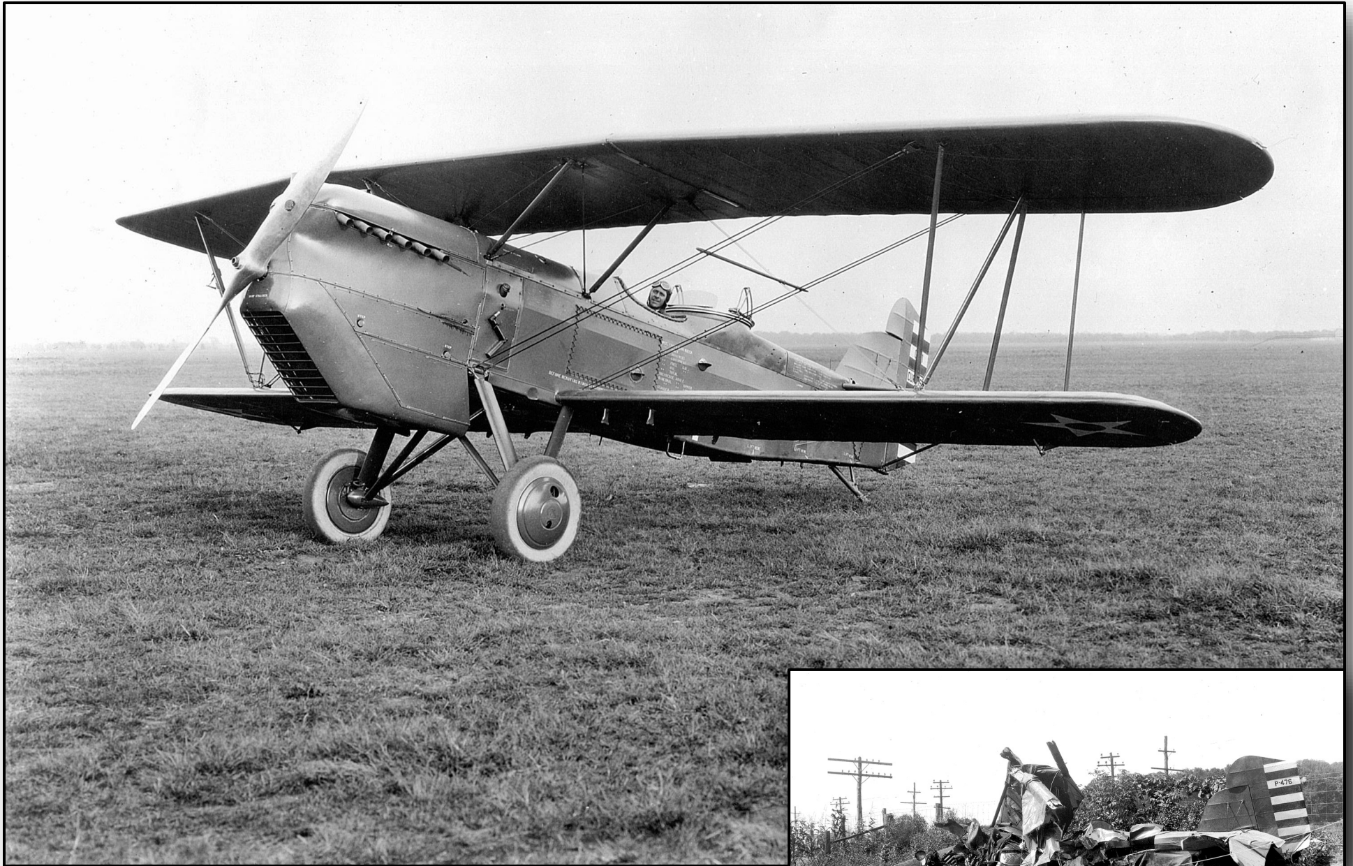
Top: Curtiss XO-1 Falcon pictured on 7 October 1927 with a Liberty engine. Right: Wreck of the Falcon on 4 September 1929, flown by Lt. George Schulgen, who was saved by his parachute, qualifying him for the caterpillar club. The crankshaft of the Liberty engine broke causing the propeller to fly off near Columbus, Ohio.
