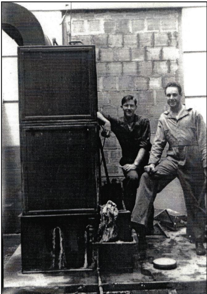
Fig. 12. SIGSALY's air conditioning system<sup>23</sup>
