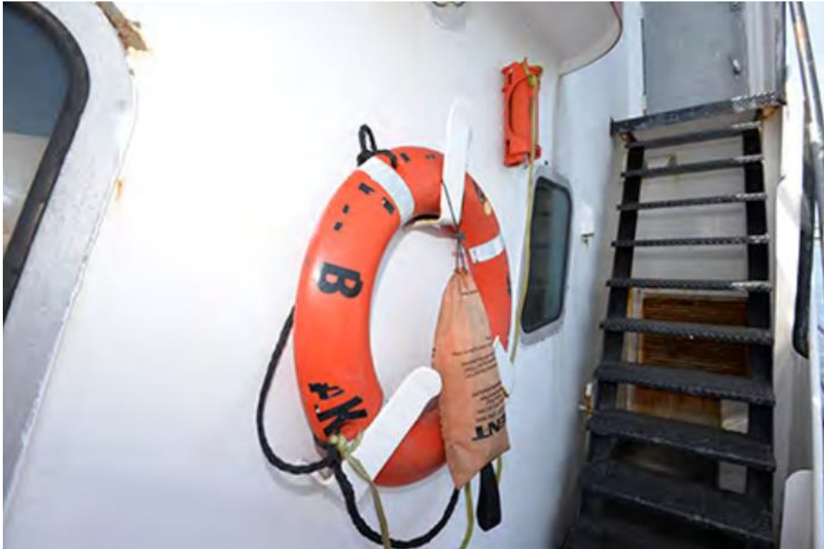
Figure 9: Engine room vent shown behind pilot house stairs from ref (p)
