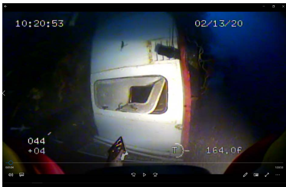
Figure 9: A man door located at the starboard stern of the accommodation suffered damage.
