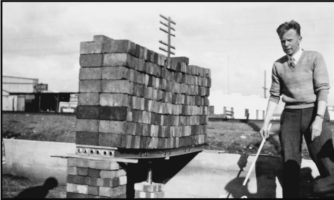
John Northrop put in many long hours during construction of the Model 1. He is shown here performing load tests on the horizontal stabilizer.
