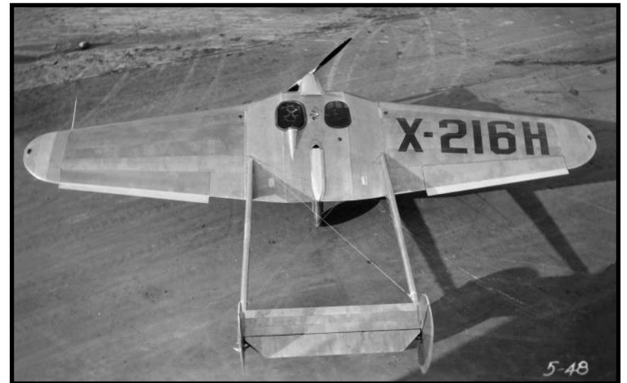
The final configuration of the Model 1 showing the uncovered right cockpit. Control wheels installed in both cockpits allowed the aircraft to be flown from either side.
