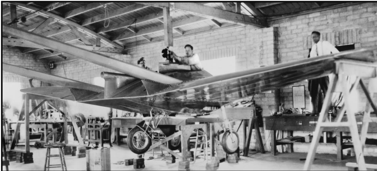
The Model 1 being suspended from the ceiling for weight and balance calibrations.
