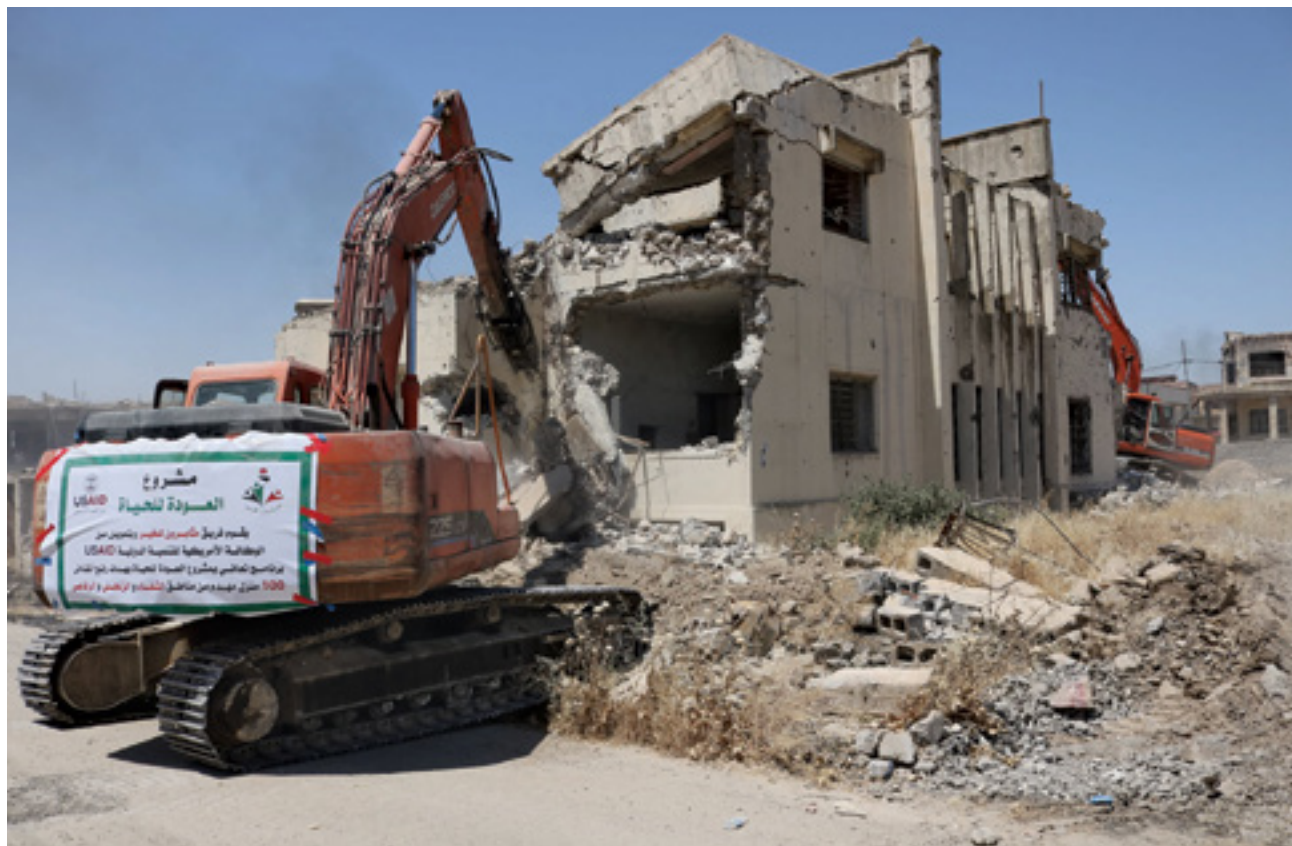
Rubble and debris are removed from demolished homes in neighborhoods in Mosul. (USAID photo)
