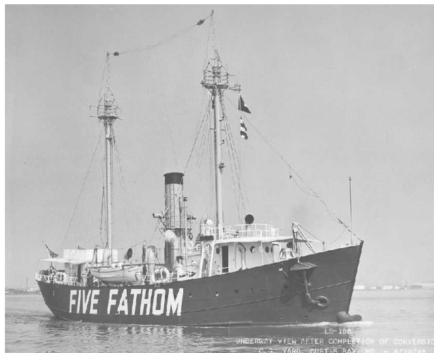
Original caption: LS-108 underway view after completion of conversion, C.G. Yard, Curtis Bay, MD., 6/29/45. LIGHTSHIP NO. 108, again refitted in 1945 for duty as a lightship on Five Fathom Bank." Photo No. 821-2; 29 June 1945; photo by H. Davis.
