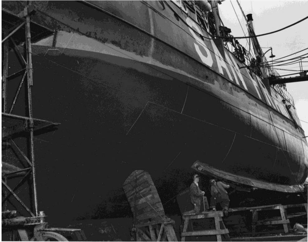
FIGURE 10. This image depicts the bilge keel of a steel lightship constructed in 1904. (Photo courtesy of the USCG Historian's Office Archives, Box 24, Washington, DC.)
