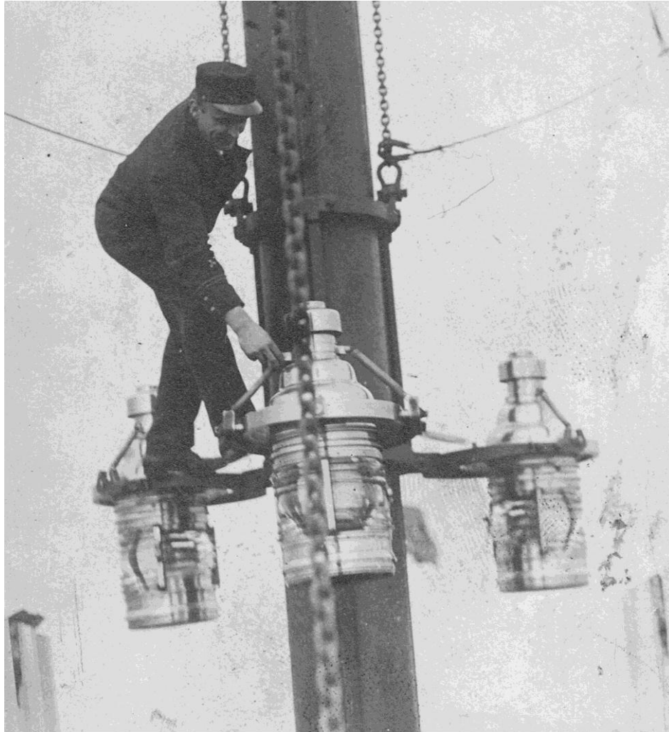
FIGURE 33. The lighting apparatus on LV3 , stationed off Shovelful Shoals, Massachusetts. The 1892 Annual Report of the Light-House Board claims that a set of 3 lanterns with brackets, gimbals, lamps, etc., weighs about 700 pounds and costs $620 (The Light-House Board 1892:30). (Photo courtesy of the USCG Historian's Office Archives, Box 25, Washington, DC.)
