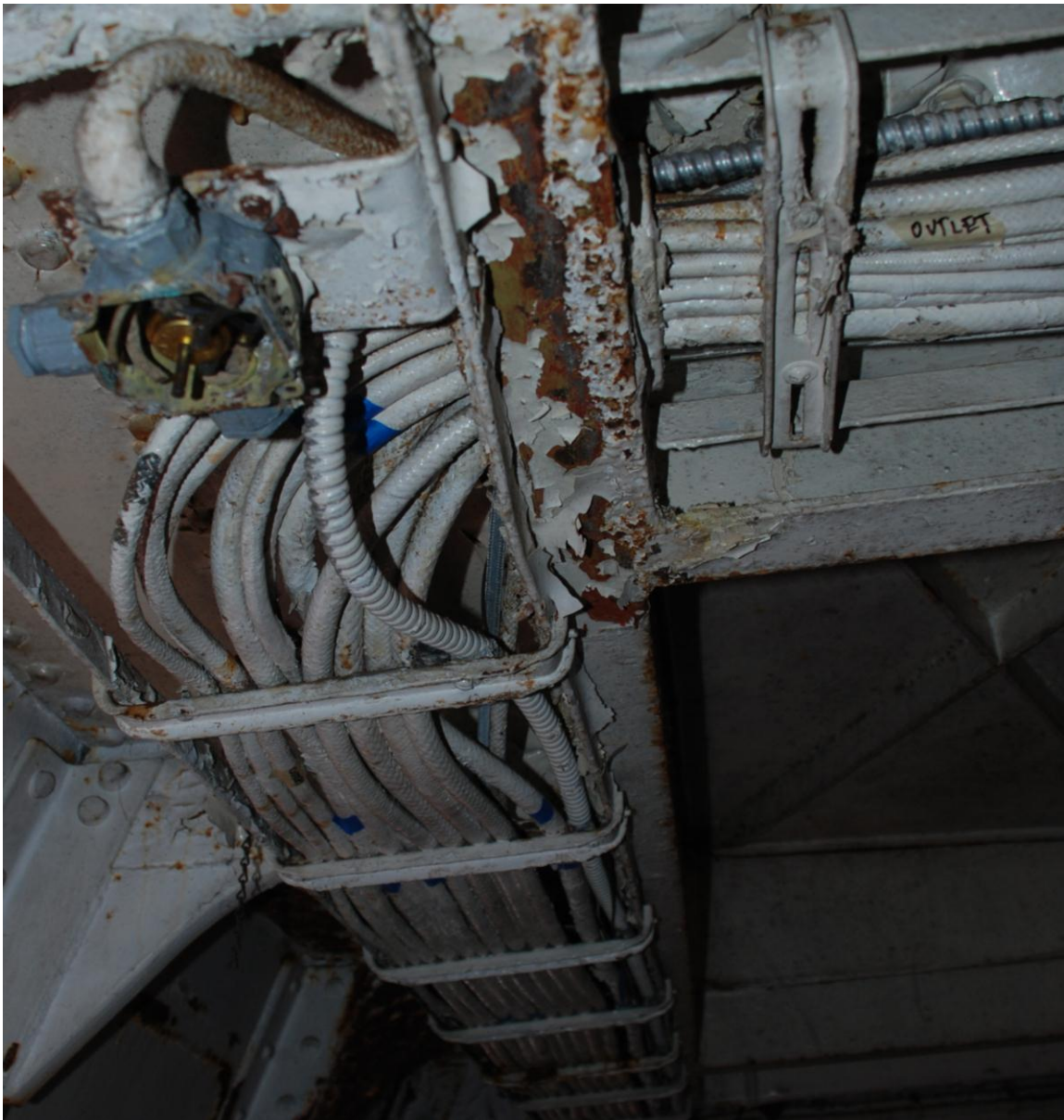
FIGURE 50. Electrical wiring cables onboard LV83 . Grouped together and painted white, tape was required to prevent confusion while tracing wires. (Photo by author, 2010.)
