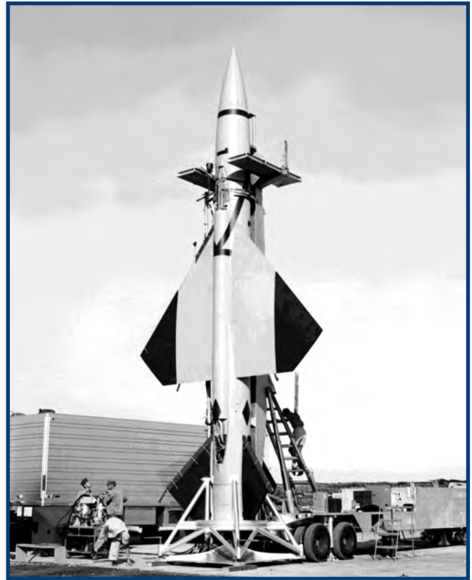
Top: First flown in 1952, the Boeing BOMARC ( BO eing Mi chigan A erospace R esearch C enter) originally carried an F-99 designation, but this changed three years later to IM-99. The XF-99 shown above had the vertical stabilizer on the bottom and did not yet incorporate the ramjet engines for cruise flight.
