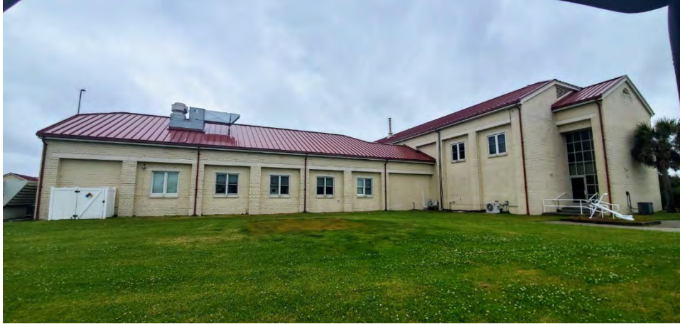
Photograph 7. Multi-Mission Building, west and south elevations, facing northeast (USCG 2020)
