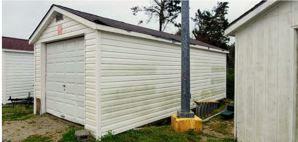
Photograph 14. PW Lawn Maintenance Shed #2, northeast and northwest elevations, facing south (USCG 2020)
