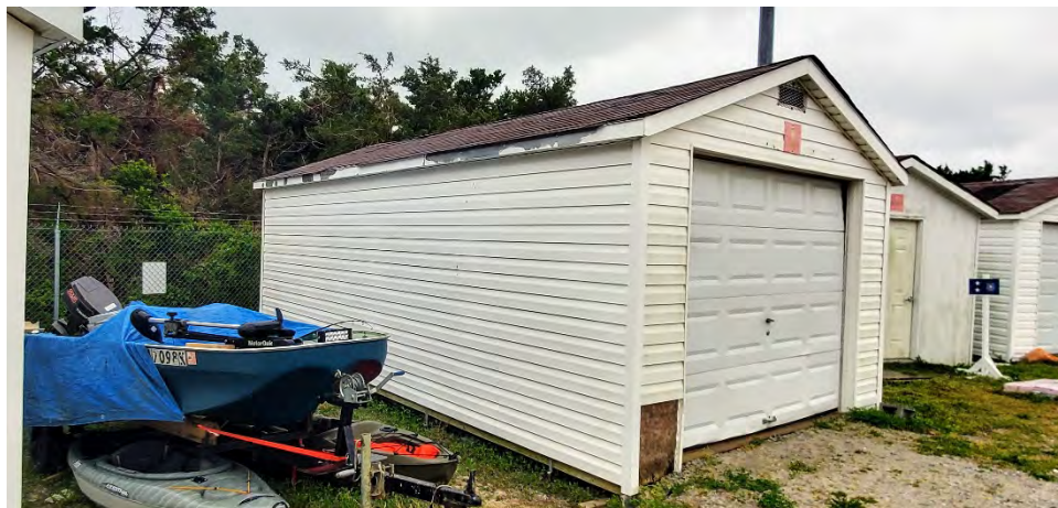
Photograph 15. PW Lawn Maintenance Shed #2, southeast and northeast elevations, facing west (USCG 2020)
