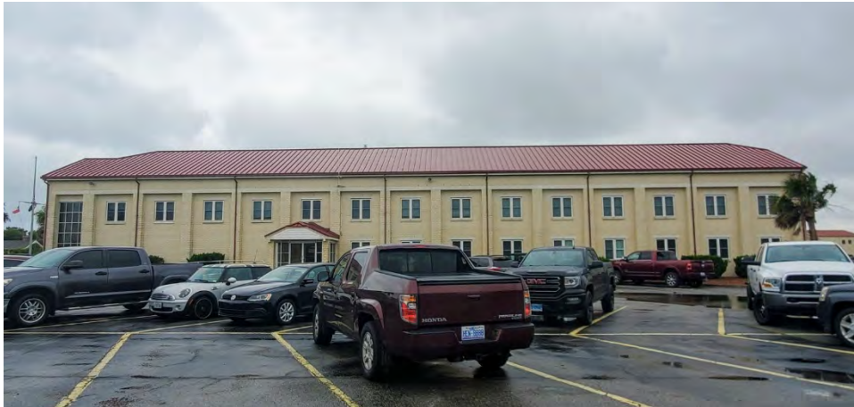
Photograph 8. Multi-Mission Building, east elevation, facing west (USCG 2020)
