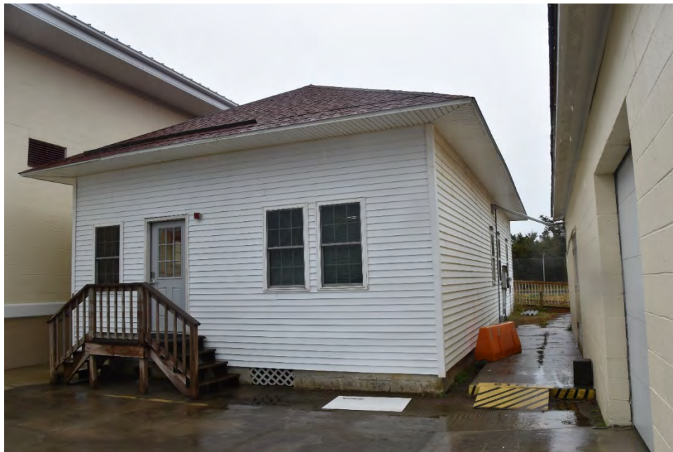
Photograph 12. ISD Office, west and south elevations, facing east (AECOM 2020)
