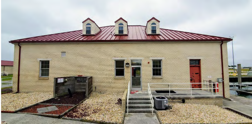
Photograph 4. Prevention Building, east elevation, facing east (USCG 2020)
