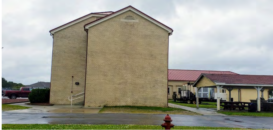
Paragraph 10. Multi-Mission Building, north elevation, facing south (USCG 2020)
