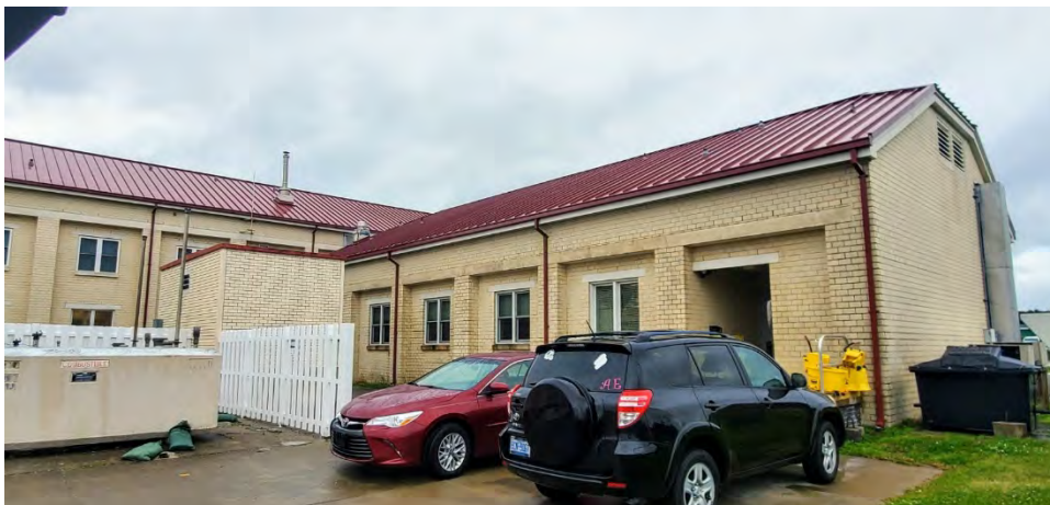
Photograph 9. Multi-Mission Building, west elevation of the main building and north elevation of the ell, facing southeast (USCG 2020)
