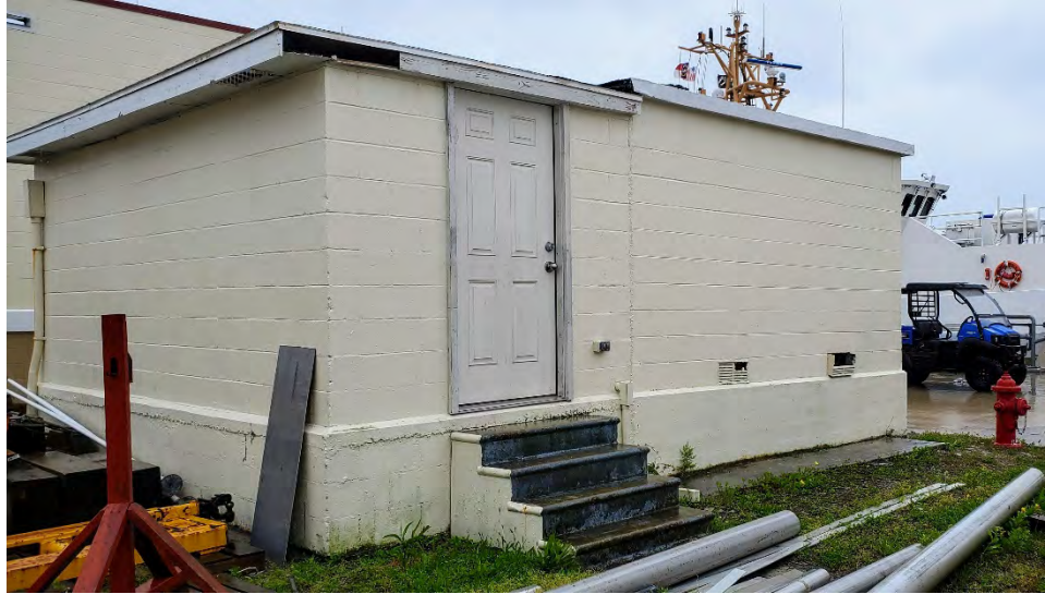
Photograph 18. Dock Side Utility Building, east and north elevations, facing southwest (USCG 2020)
