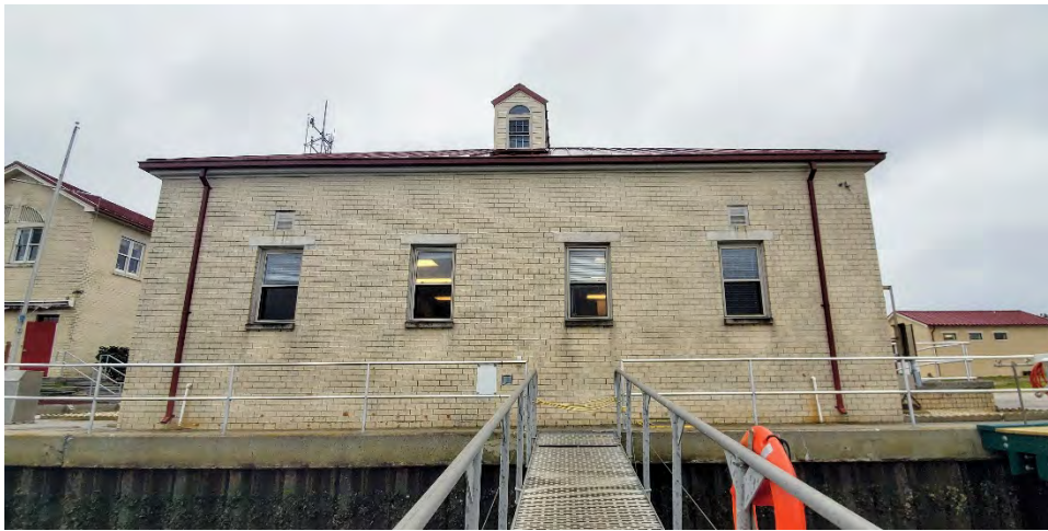
Photograph 5. Prevention Building, north elevation, facing south (USCG 2020)
