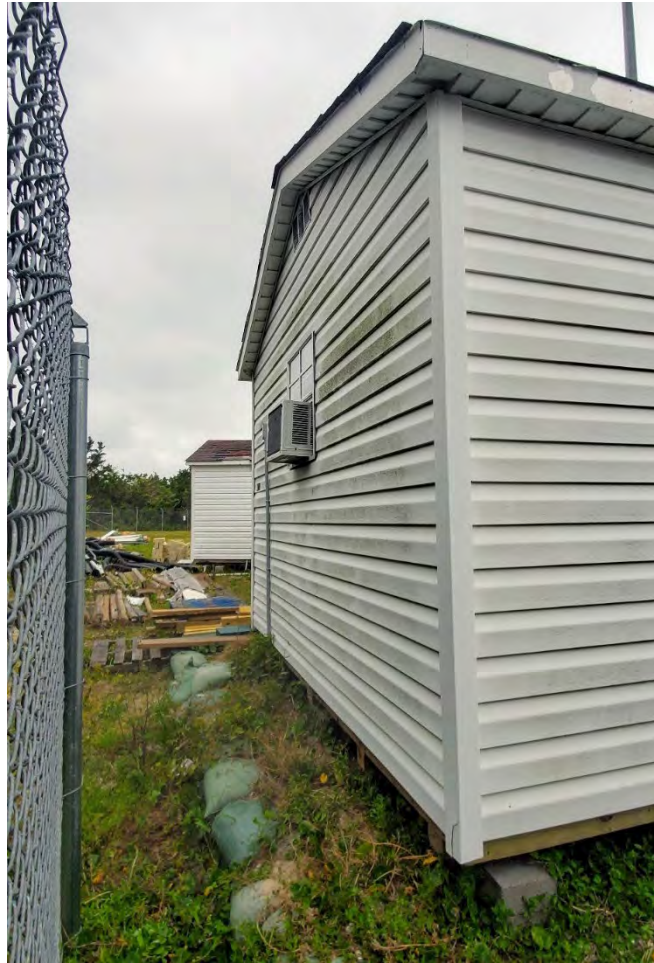
Photograph 16. PW Lawn Maintenance Shed #2, southeast and southwest elevations, facing northwest (USCG 2020)
