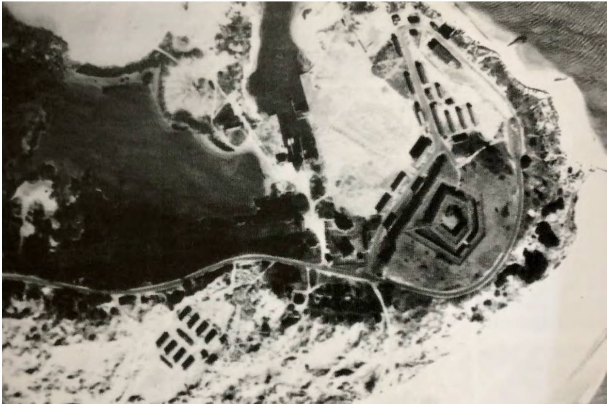
Figure 3. Aerial view of USCG Station Fort Macon and historic Fort Macon, in 1945 (Branch 2013)
