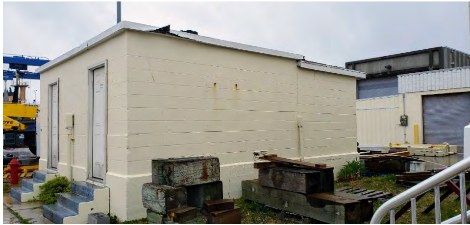
Photograph 17. Dock Side Utility Building, west and south elevations, facing northeast (USCG 2020)
