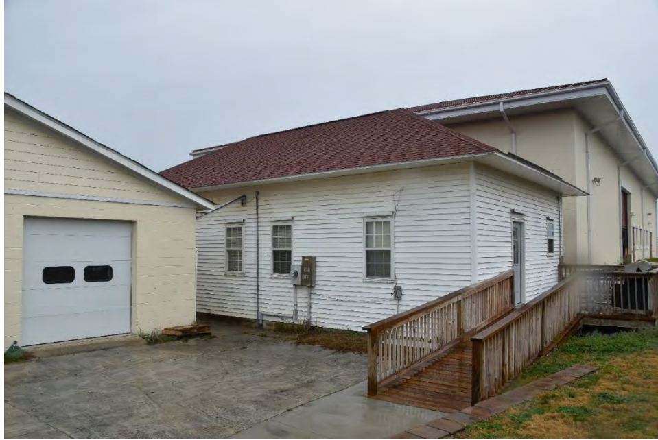
Photograph 13. ISD Office, south and east elevations, facing northwest (AECOM 2020)
