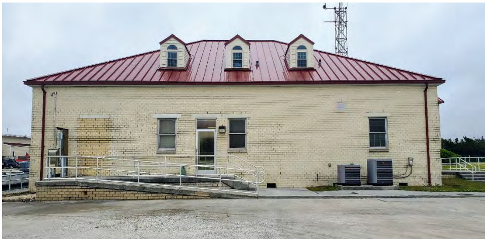
Photograph 6. Prevention Building, west elevation, facing west (USCG 2020)
