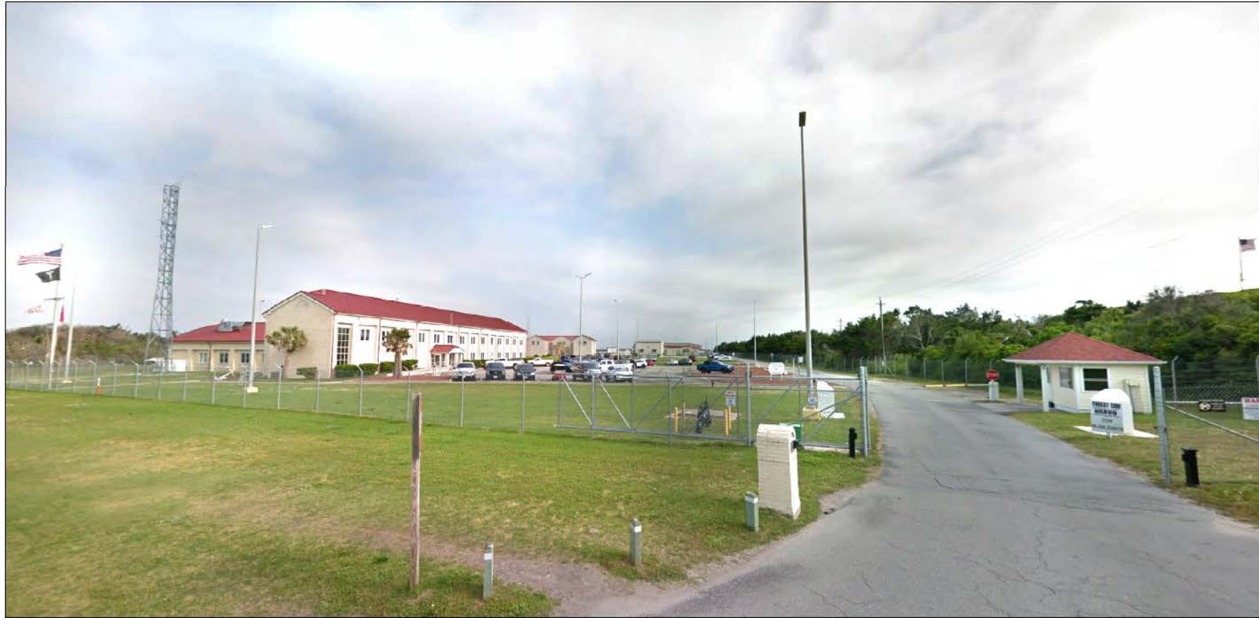
USCG SECTOR FORT MACON ENTRANCE STREET VIEW - EXISTING
