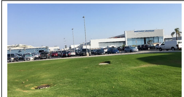
The project site is located immediately adjacent to the south of an existing surface parking lot (shown above) and currently functions as a stormwater detention basin that collects surface water runoff entering from an underground double box culvert.
