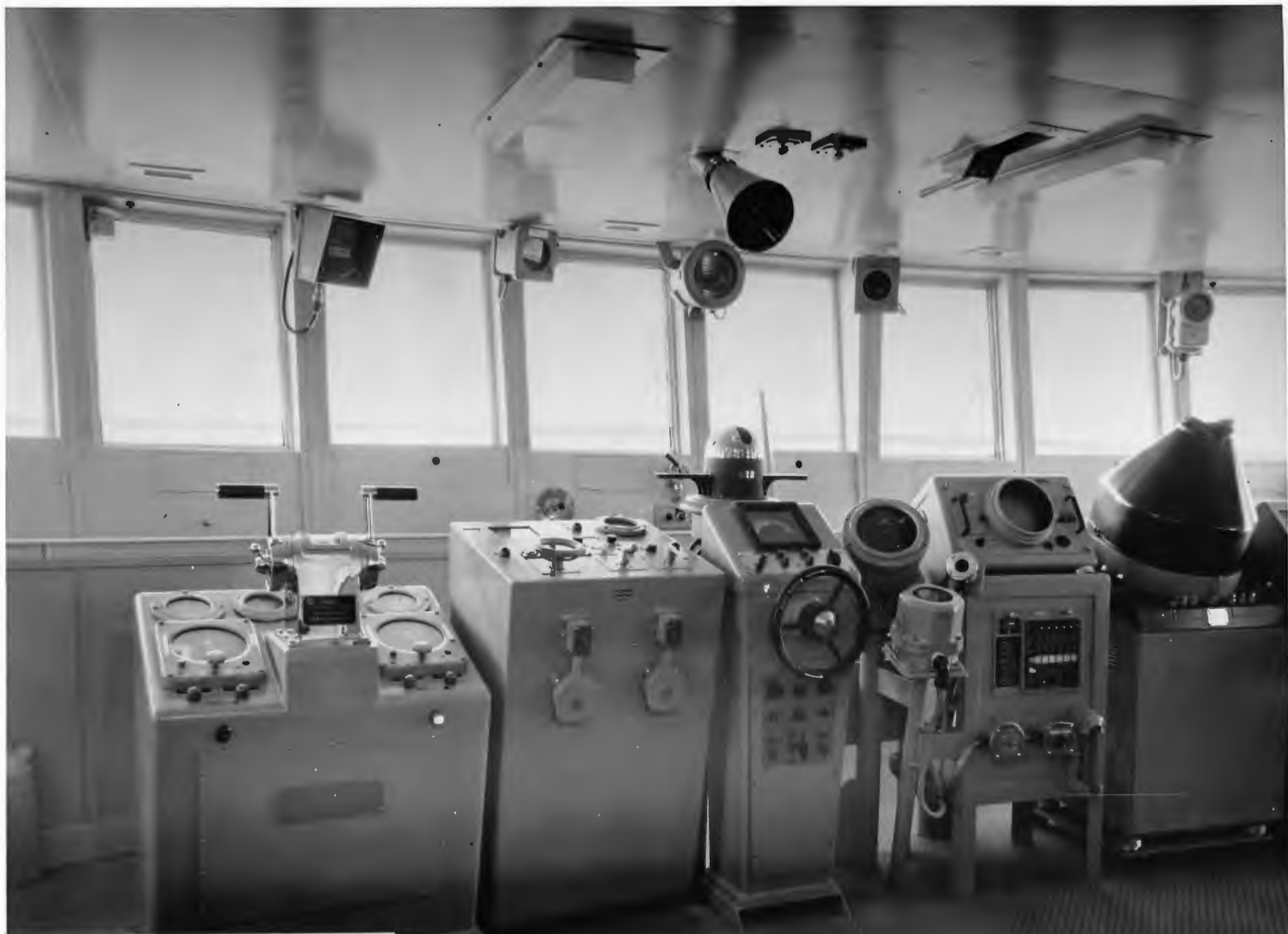
U.S.C.G.C. HAMILTON AVONDALE SHIPYARDS, INC. PILOT HOUSE ( LOOKING FWD) 2/18/67 NEG. NO. 7-546
