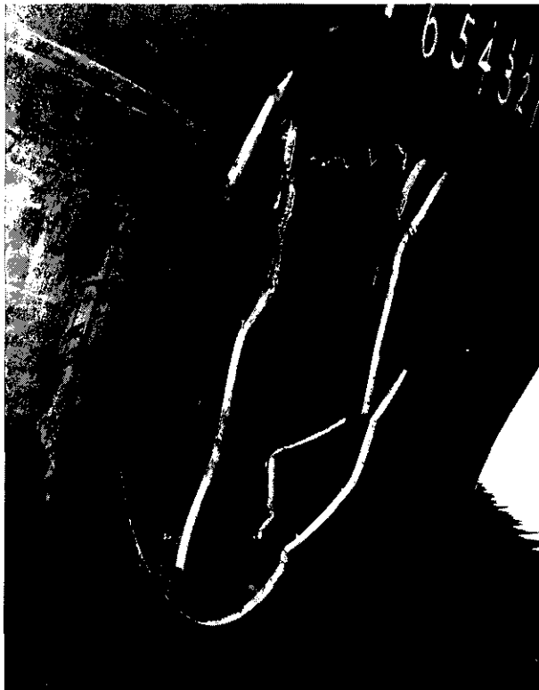
Figure 10. WIND Class shell structure damage
