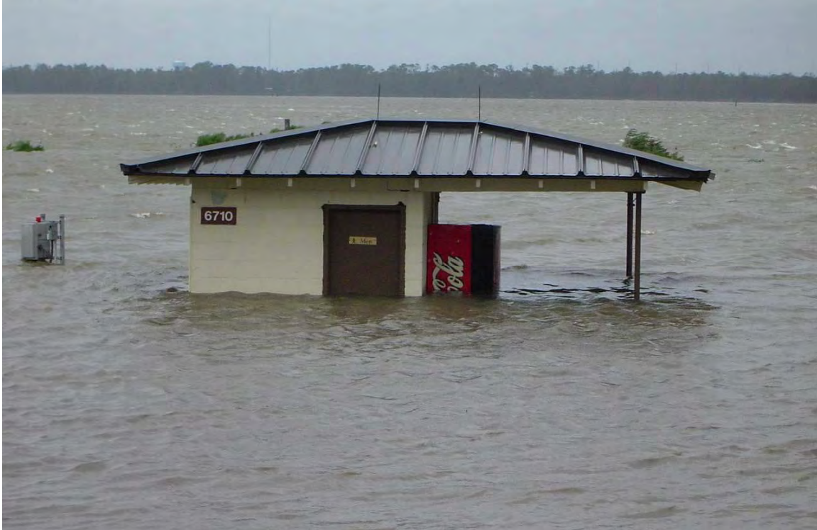
Hurricane Katrina's record low pressure, 125 mph winds and high tides converged to create a storm surge that raised the level of the Back Bay of Biloxi nearly 30 feet above normal. This restroom lies between the 12th and 13th holes on the Keesler AFB golf course (USAF photo).
