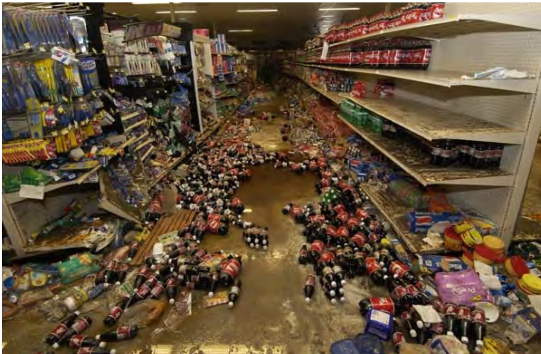
Several feet of water from Hurricane Katrina’s storm surge inundated the commissary and base exchange, wrecking the contents and necessitating a careful cleanup project.
