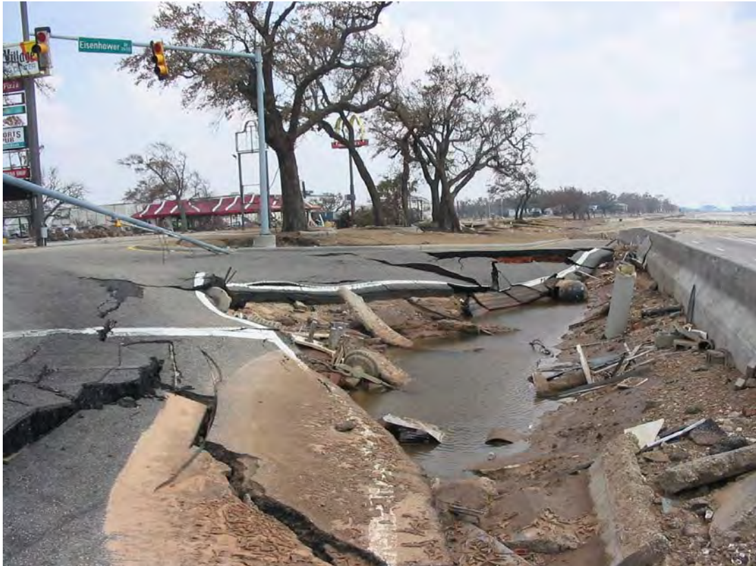
The damage from Hurricane Katrina made many roads around Keesler AFB impassible, even after workers had cleared debris from shattered houses and downed trees. In the distance, only a roof and vertical supports remain of a fast-food restaurant.
