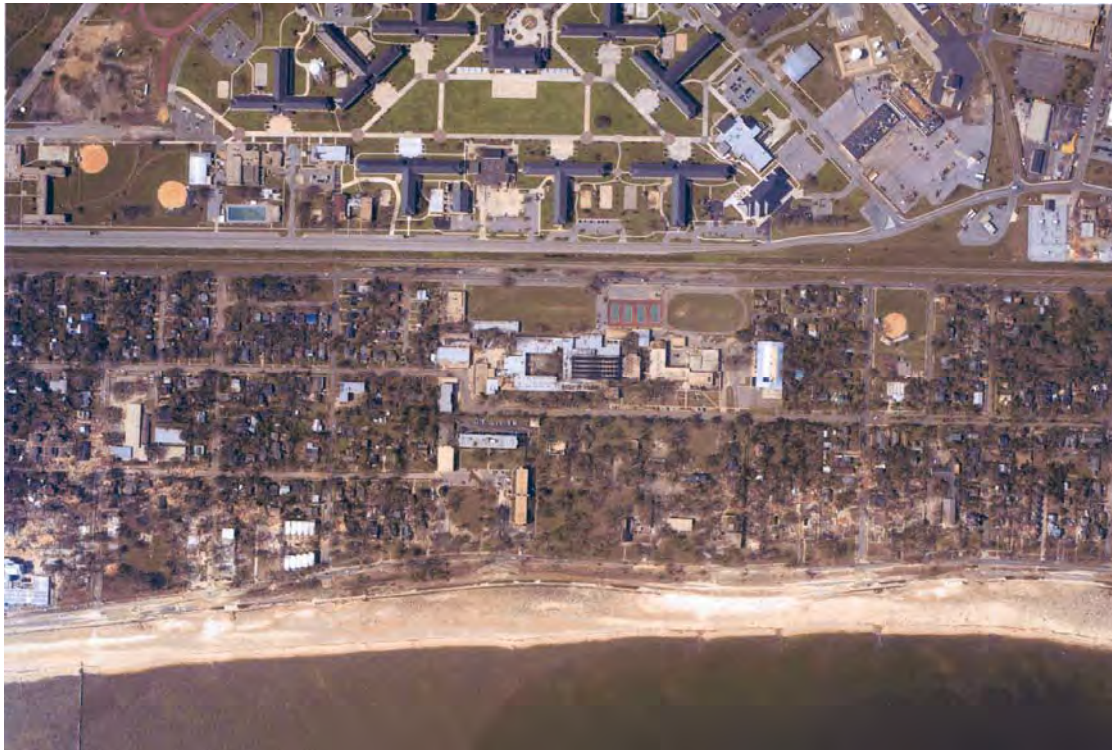
This photo, an aerial view of Keesler AFB, Mississippi, taken after Hurricane Katrina, shows the Triangle Dormitory area, which was high enough in elevation to avoid the 19-foot storm surge that devastated the residential areas just outside the gates.
