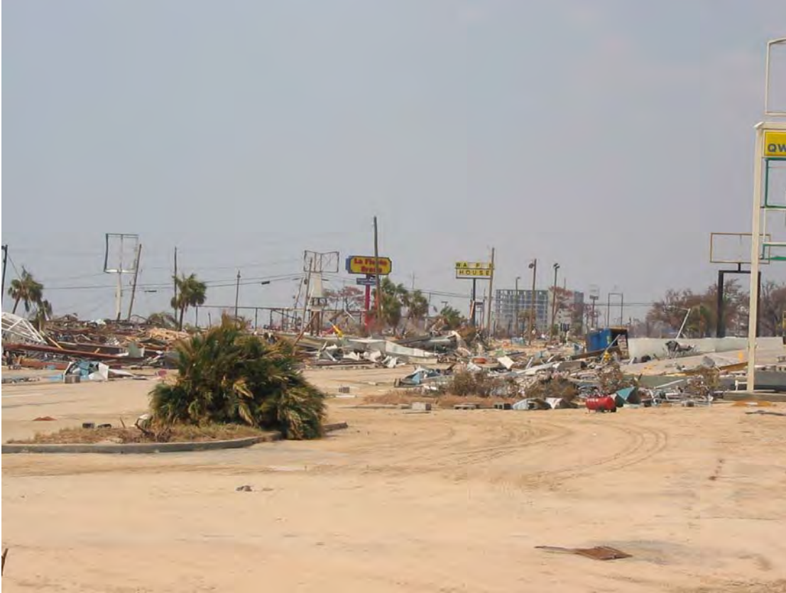
The storm surge from Hurricane Katrina devastated businesses along U.S. 90, the highway that passed through the coastal communities near Keesler AFB, Mississippi.
