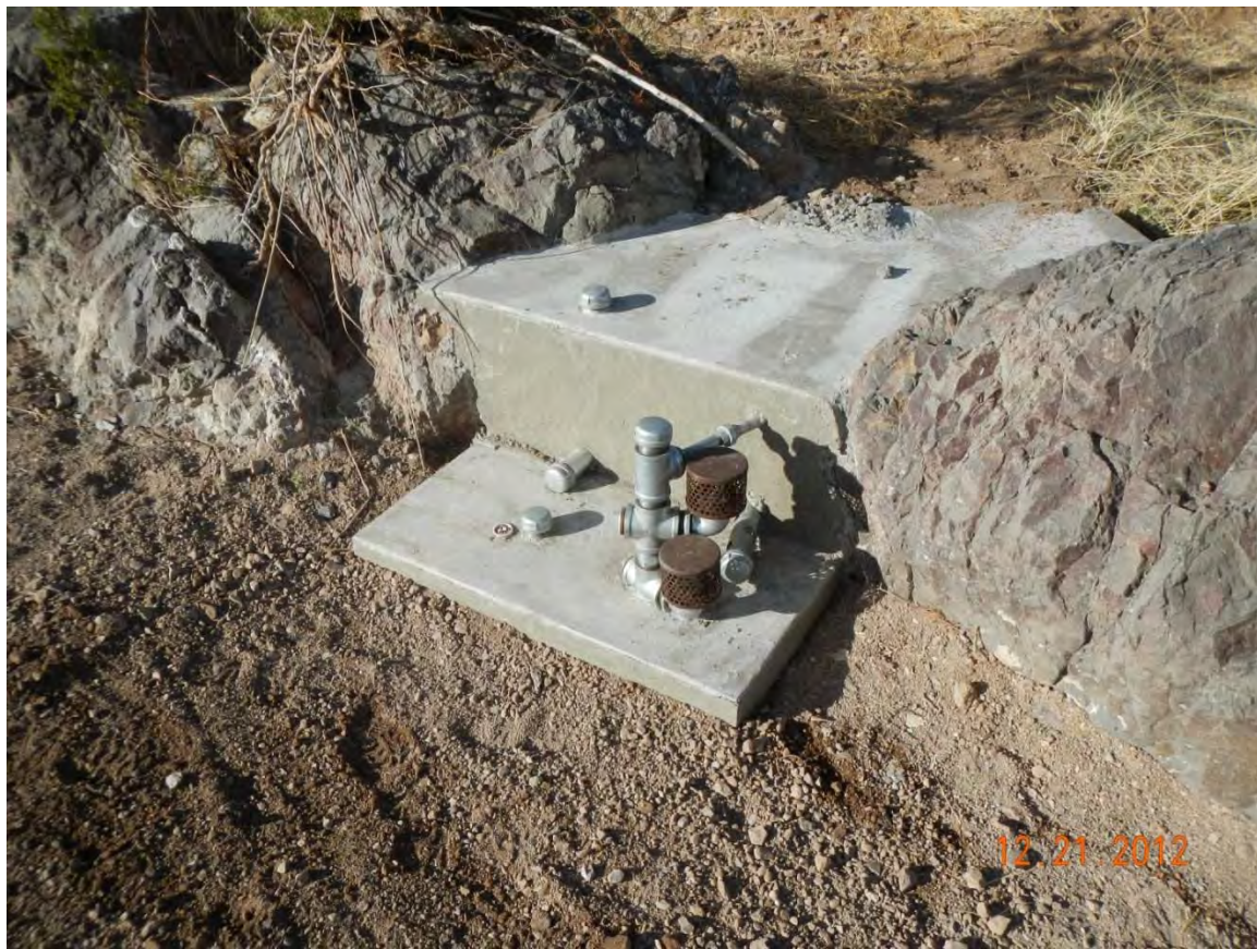
Figure 4. Float Switch Foundation (Barrel Canyon installation)
