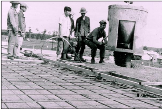
Campbell teaching about placing roof concrete
