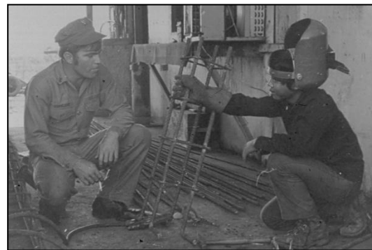
Copeland instructing trainee in welding rebar
