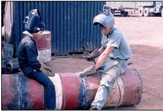
Left: Trainee and Grethey welding 55-gallon drums for culvert material
