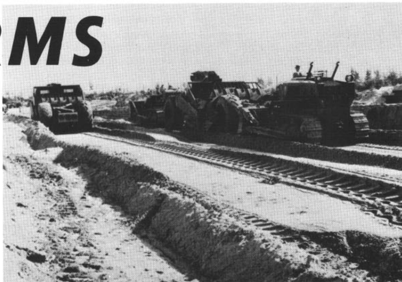
DIG THIS —Heavy equipment operators move earth for runway.
