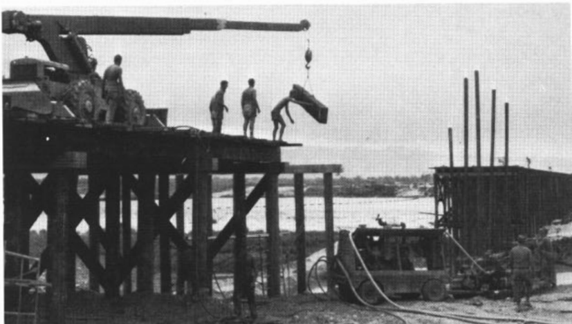
A LONG ONE —Seabees build 2040-foot bridge southwest of Da Nang.
