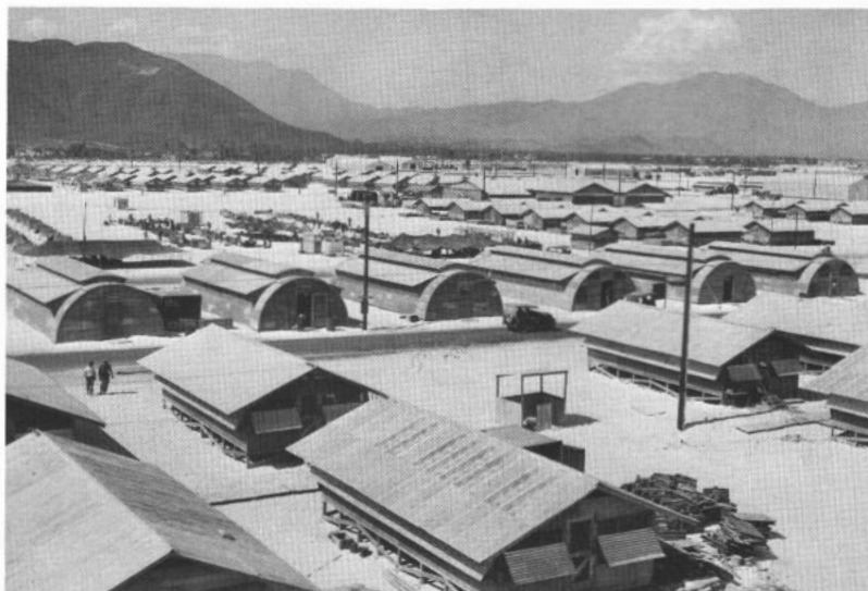
SEABEE CITY —Small part of CB-built facility at Red Beach.
