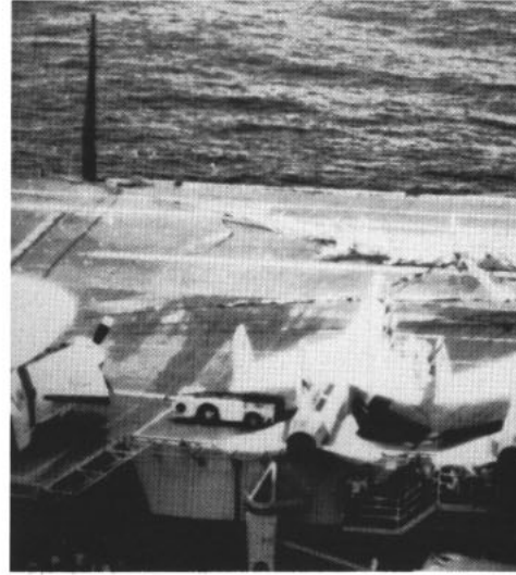
HOME SAFE— Crusader with stuck landing gear makes barricade arrested landing aboard Ticonderoga (CVA 14).
