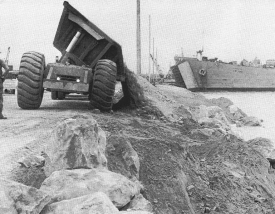
SHORE LINING —MCB Forty builds all-weather cargohandling facility at Chu Lai.
