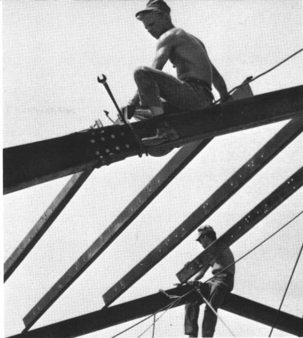
RT: Steelworkers finish off a Butler building frame.
