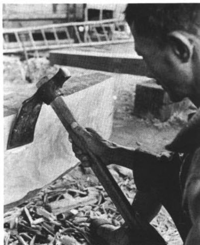
PLANER —Vietnamese junk builder finishes scarf joint of sao wood.
