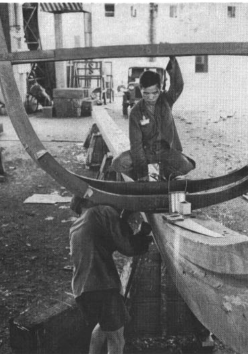
STARTING POINT —First ribs are placed on keel. Below: LT R. J. Pratte, USN, checks out rib frame.
