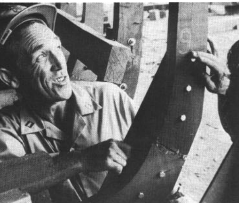
PLANER —Vietnamese junk builder finishes scarf joint of sao wood.
