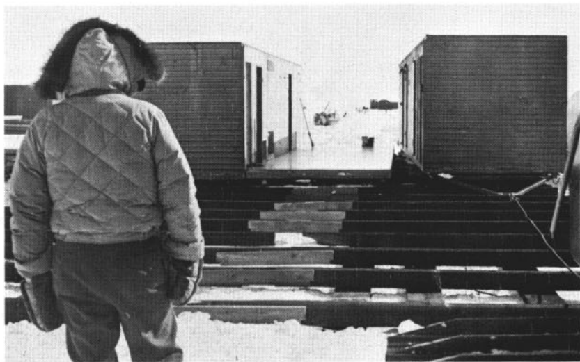
PREFABRICATED units that will comprise the station are placed on bases. Below: Station unit is off loaded after being air lifted 1400 miles from McMurdo.
