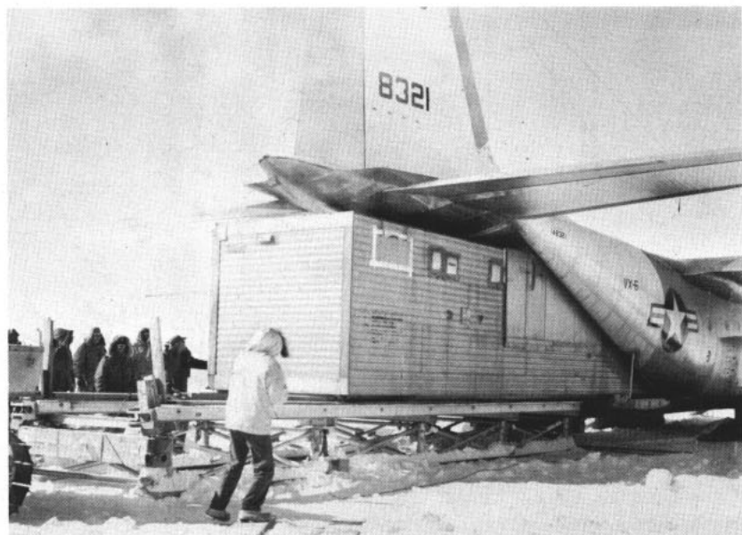
PREFABRICATED units that will comprise the station are placed on bases. Below: Station unit is off loaded after being air lifted 1400 miles from McMurdo.
