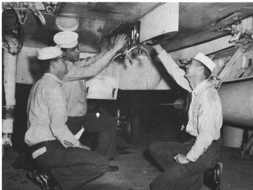
SQUADRON's aviation ordnancemen check bomb rack on A4C Skyhawk.
