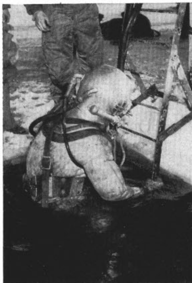
SLIPPING beneath freezing water, diver must walk under ice to work site. He can stay only a few minutes.
