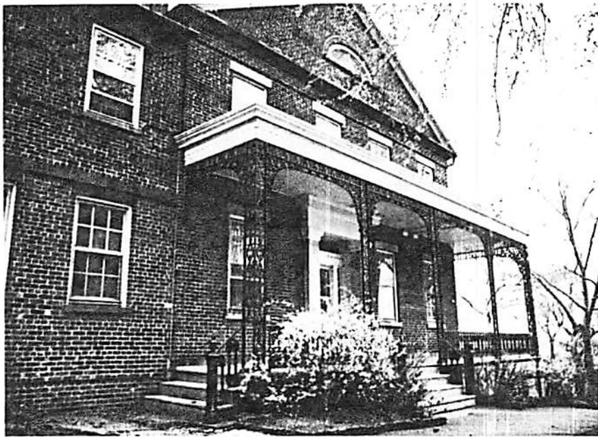
Building 135, showing intricate wrought iron work
