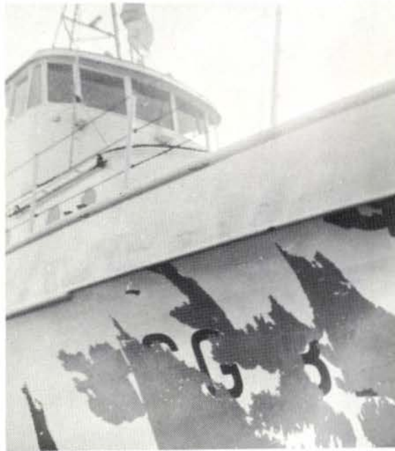
Failure of high quality coating due to application over dirt contaminated surface. Official Coast Guard photograph.
