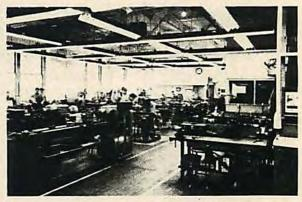
Where ceilings are high, efficient illumination may require direct light with the type units illustrated. Photographs, courtesy General Electric Company.
