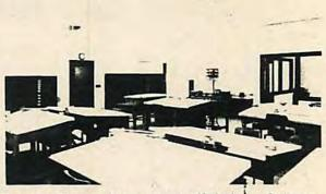
Semi-indirect fluorescent lighting fixtures create a bright overhead. Illumination is both direct and indirect—assuring clear visibility of three-dimensional objects.
