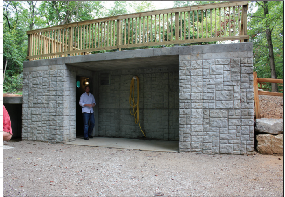
A new safe room replaced the former outdoor safe room — a buried metal culvert — at Theodore Naish Scout Reservation near Bonner Springs. The new safe room was constructed with mitigation grant funding.
