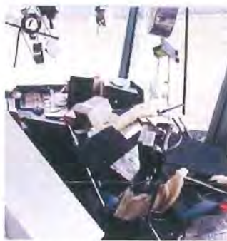
Damage to the control tower at Sea-Tac Airport, 2001 Nisqually magnitude 6.8 earthquake.***
