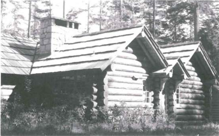
The log cabin near the old entrance, pictured in the late 1930s. Notice the large shakes on the roof, and the natural color of the oiled logs.
