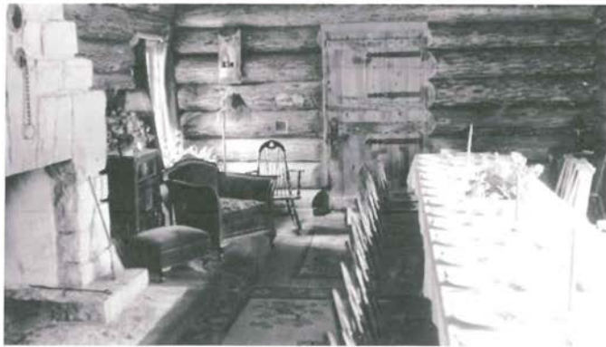
The interior of the cabin, set up for a formal dinner in the 1930s. The rock fireplace is on the left, and front door is on the back wall.
