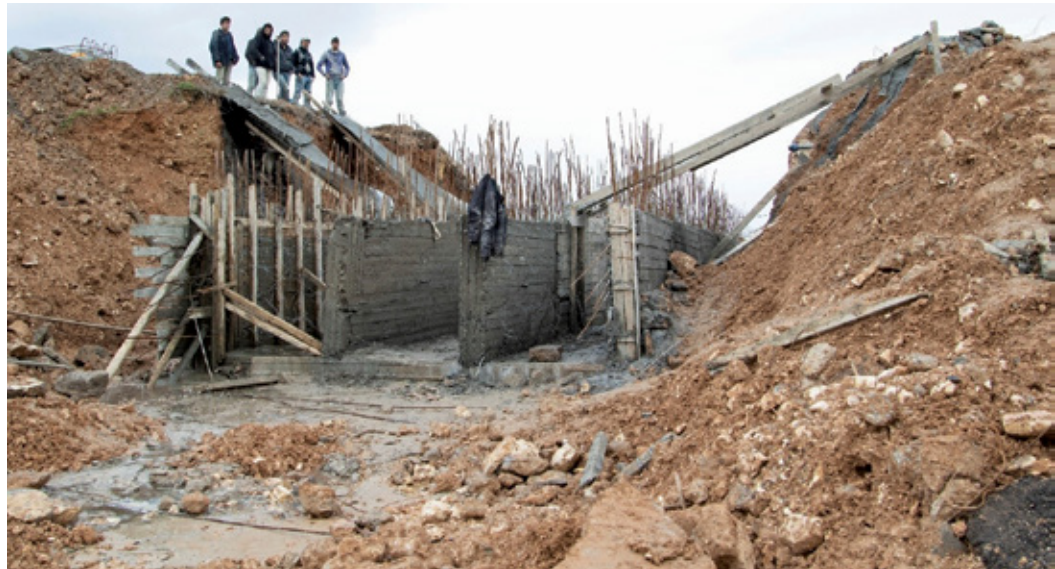
Local Syrians stand over the ruins of a bridge destroyed by ISIS in northern Syria. (U.S. Army photo)
