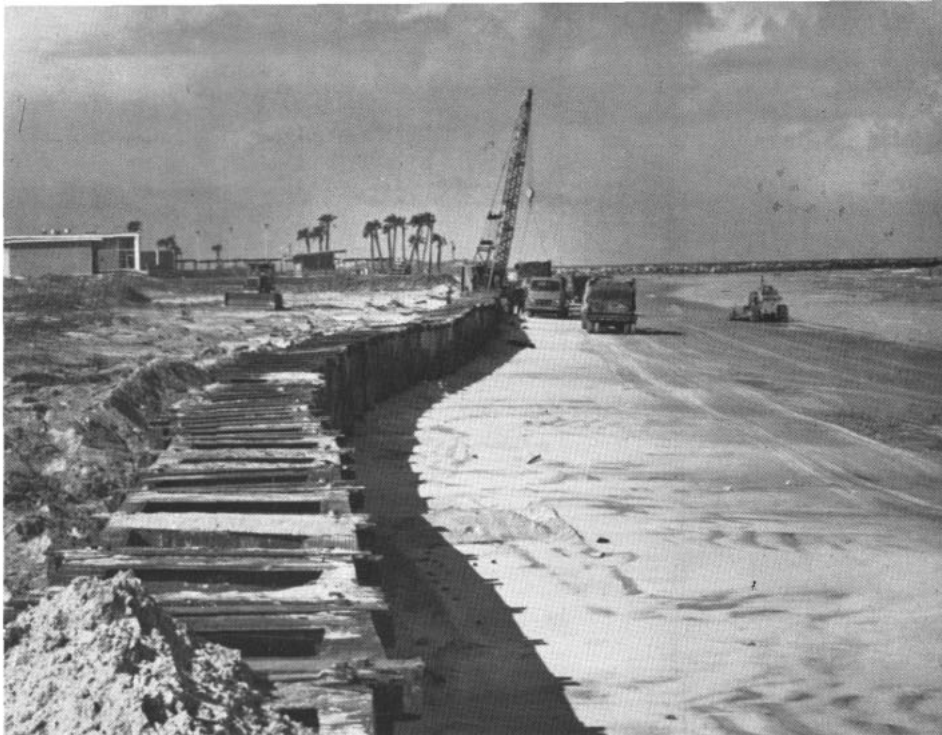
BEACH PARTY —Seabees place pontoons along shore to form barrier. Left : Steelworker cut holes in top of pontoons.
