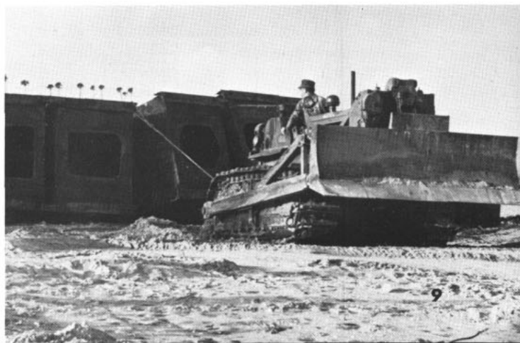
LOTS OF PULL —Cat skinner pulls pontoons from bay with dozer ( rt ) and crane lines up sea wall on eroded beach.
