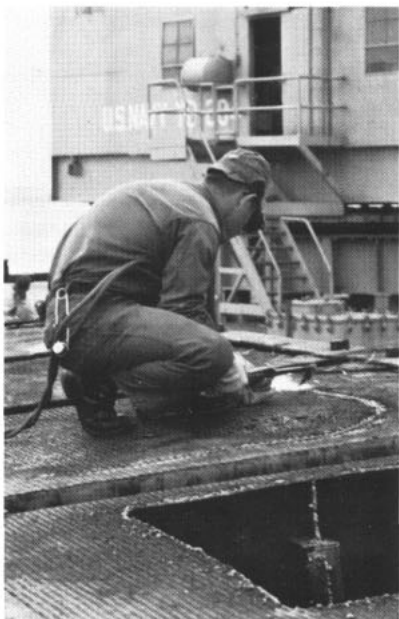
BEACH PARTY —Seabees place pontoons along shore to form barrier. Left : Steelworker cut holes in top of pontoons.
