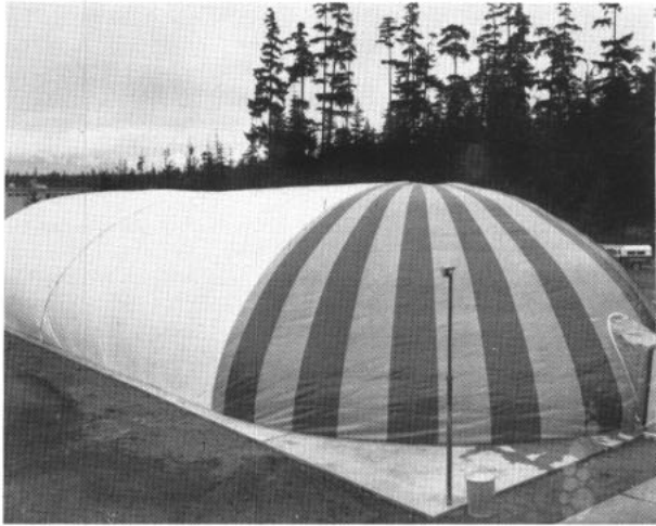
ALL-YEAR SWIMMING pool at Naval Ammunition Depot, Bangor, Wash., is covered by economical, heated air house.
