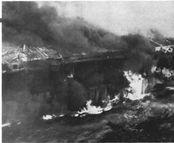
INFERNO AT SEA —Leaking gasoline and ammunition caused explosions, making damage control difficult.
