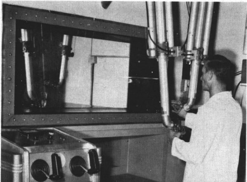
MECHANICAL hands do 'hot' experiment at NRL's Nuclear Reactor Facility.
