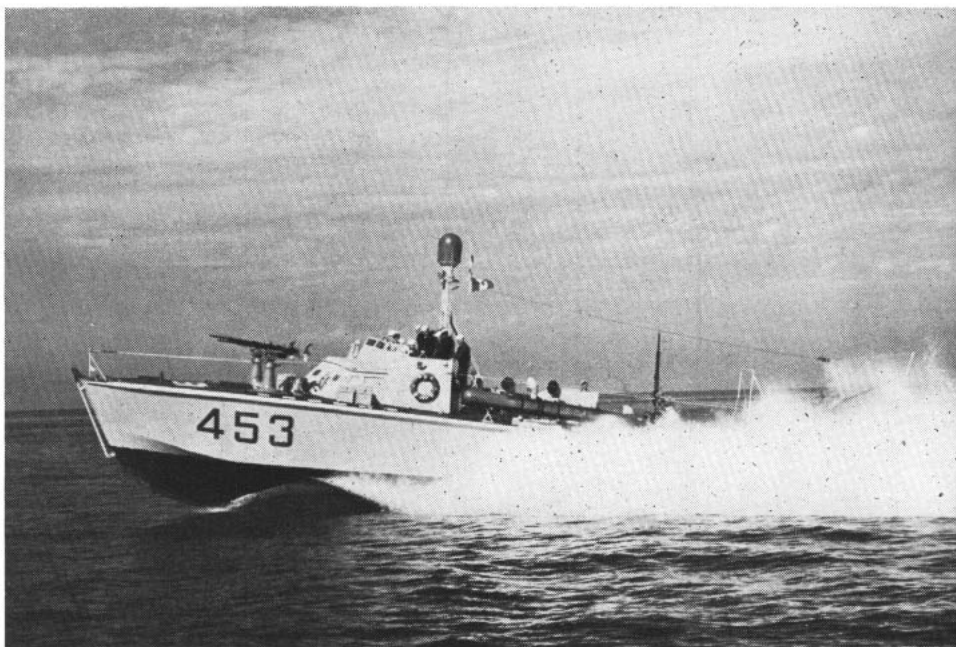
SURFACE SKIMMING — Motor torpedeo boat 453 speeds by at operational speed of 32 knots which allows a cruising range of approximately 100 miles.
