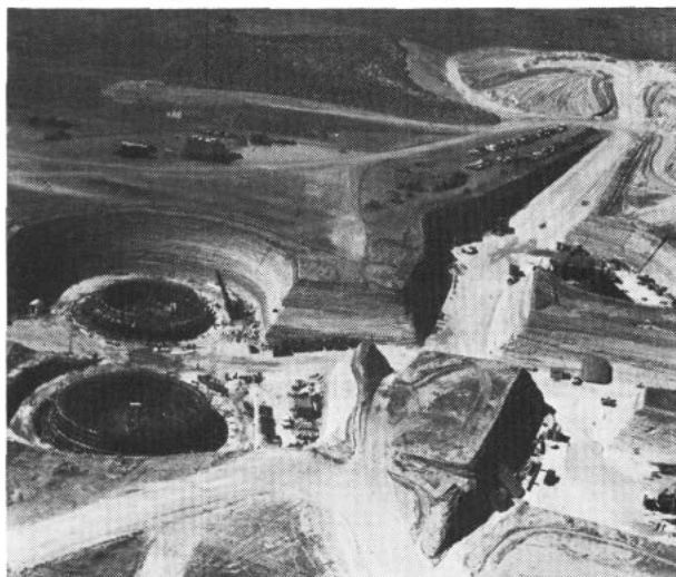
DIG THIS —Army engineers dug this area near Denver, Colo., in building underground USAF Titan missile sites.
