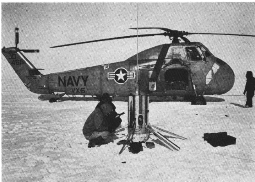
ANTARCTIC GRASSHOPPER —Deep Freeze personnel check Navy Grasshopper weather station that automatically transmits reports by radio signals.
