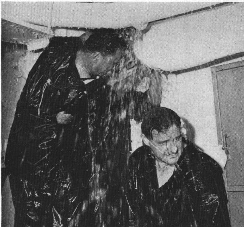
DRENCHED damage controlmen work in spurts to stop leak in Buttercup's ruptured water line. Before it's fixed trouble will break out elsewhere.
