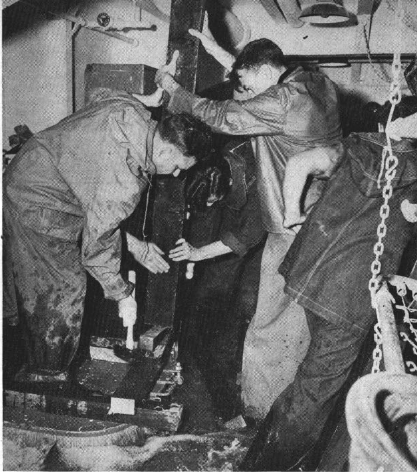
SHORES are set up to seal a hatch sprung by blast from below (above). Center: Men check a hole made by a bomb in deck of living compartment.
