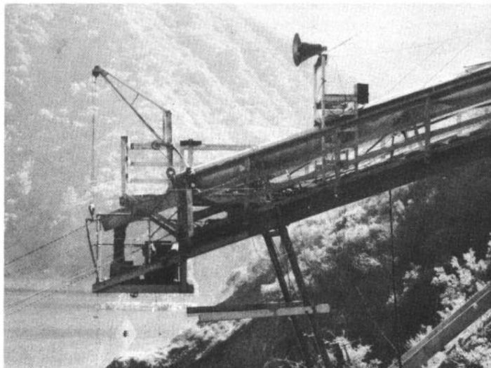
REAL TORPEDO is propelled into lake (left) by giant 'pea-shooter' (right). High-speed cameras record antics of fish.
