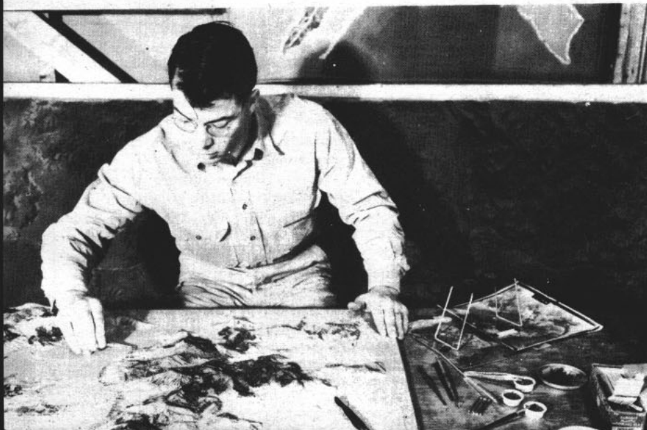
ELEVATION is shown by layers of heavy cardboard (above), which are secured with rubber cement, tacked for rigidity. Landscape details are added (below).
