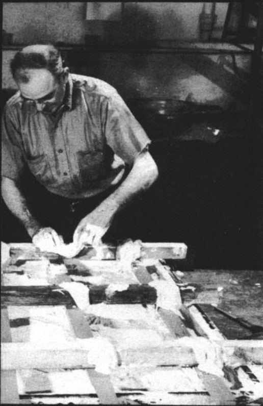
FOAM RUBBER is used in casting (above). After curing, sponge rubber relief map is pulled away from plaster negative (below). Result: perfect scale model.
