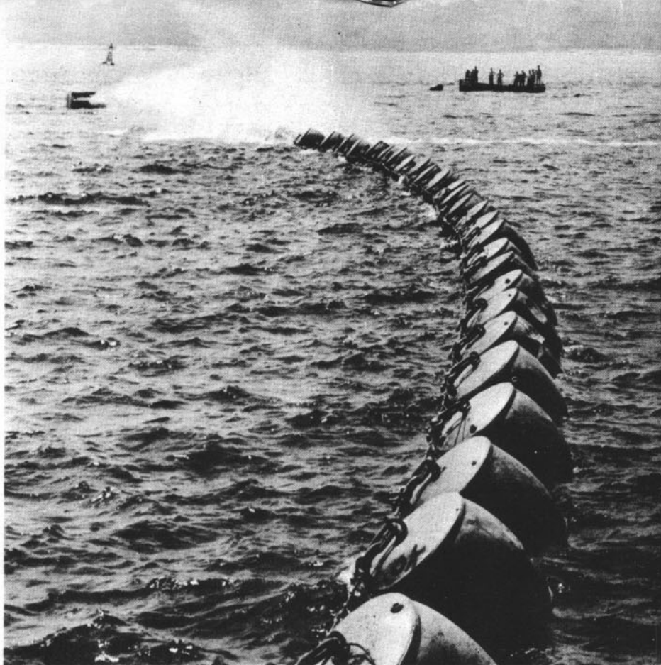
NET DEFENSES are tested against torpedoes (above). Odd-looking, horn-nosed net tender (facing page) elevates a broken section of a net. Highly-specialized maintenance work on a net line is carried out (below) in wintry north Atlantic.
