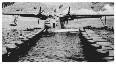
FLOATING berth for seaplanes, which can be moved out from shore to simplify mooring waterborne aircraft, developed and successfully tested by BuDocks.
