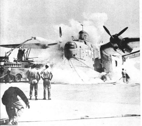
SMOKE pours from an engine of a PBM (above) as the Navy's "two-minute men" swing into action. Fog-foam equipment is being used to blanket the fire.
