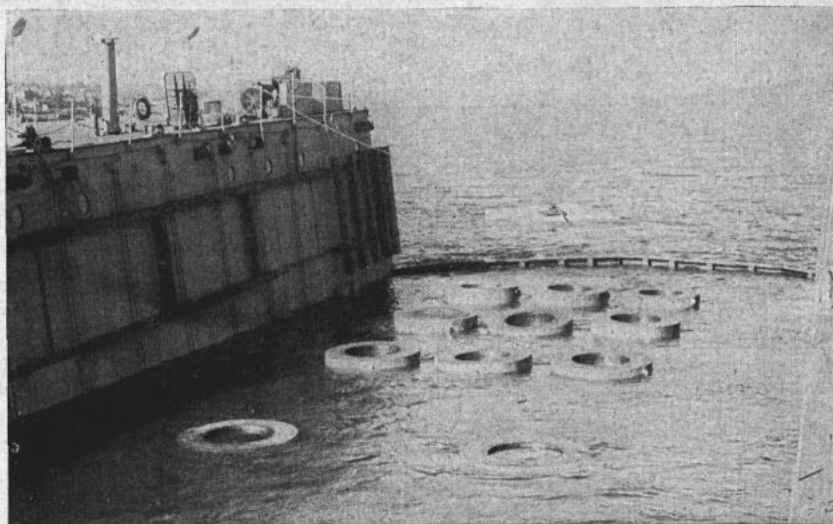
LOOKING AFT in partially submerged drydock shows shock-absorbers.
