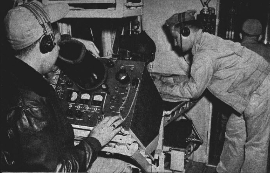
STUDENT OFFICERS in advanced training phase of ground school are checked out in the use of radar (foreground) and navigation equipment (right).
