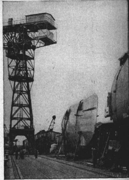
AMIDSHIPS SECTION of the German Type 21 is assembled. Equipped with
