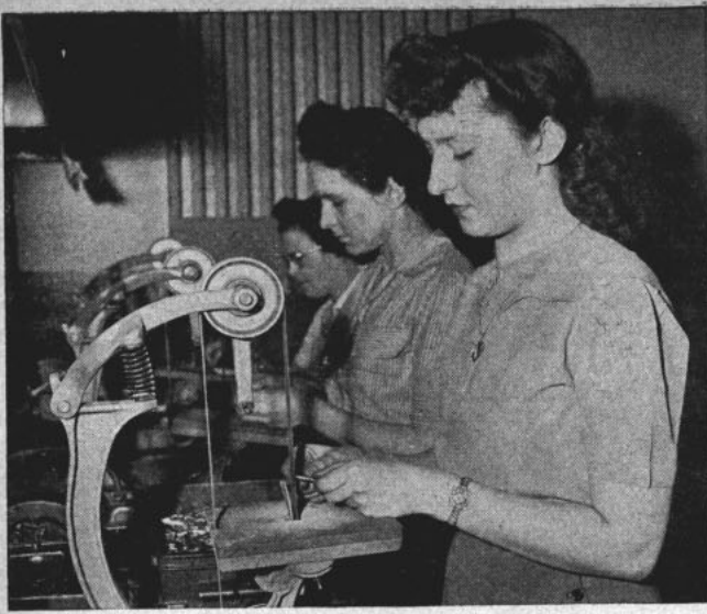
PURPLE HEARTS are smoothed (left) to a satin finish on rotating sanding strips. At right, holding rings are soldered on medals to decorate the Navy's most deserved by one of the many technicians at the Philadelphia mint.
