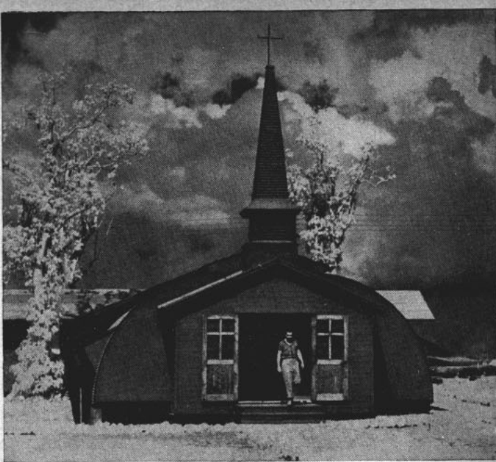
USING A QUONSET hut as a starting point, a Construction Battalion on Guam built this chapel for its own use.
