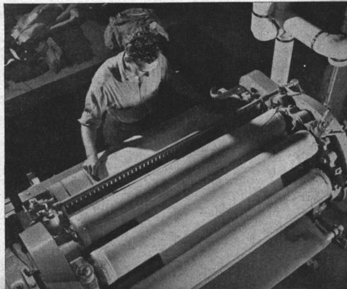
FLATWORK IRONER (below) of type used on cruisers is manned by Navy laundry school student. His mates (below, left) practice on the LST laundry unit, the smallest.
