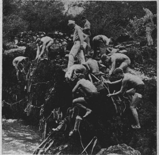
DEMOLITION CHARGES, strung together, are set in a rock beach obstruction in Hawaii during UDT training.
