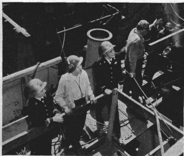
HELMETS AND SLACKS are variations in uniform of the day for Waves who board partly finished hull in Navy yard.
