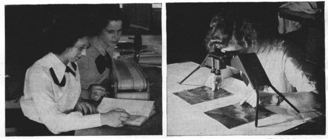
FATHOMETER recordings are checked by Waves with survey ship's records before entering on chart.
