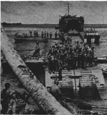
Official U. S. Coast Guard photograph Attached in sections, pontoons lay direct “roadbed” to shore.
