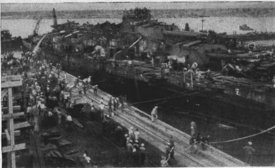
Associated Press Wirephoto UP FROM THE GRAVE: The USS Oklahoma, righted and refloated after having been capsized and sunk by the Japanese in their attack on Pearl Harbor on 7 December 1941, is shown in drydock there for further repairs.
