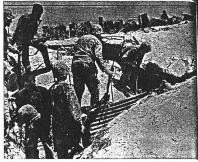
When Japs in this shelter refused surrender demand by marine at entrance, grenades ended their resistance.
