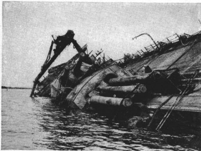
THE OKLAHOMA slowly comes upright as a new system of cable tension is utilized to raise the stricken battleship. Guns and decks are covered with barnacles.
