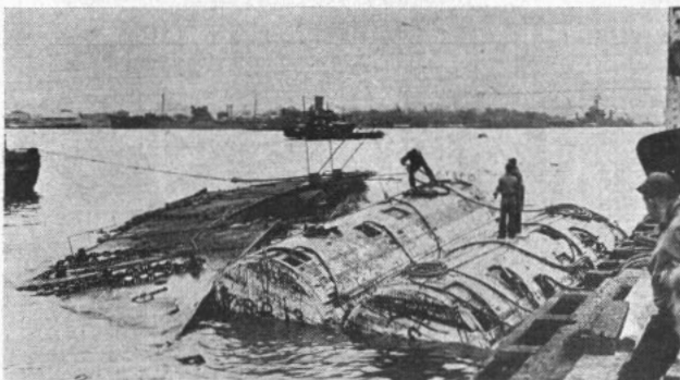
THE "OGLALA," mine layer. At left: The hull of the capsized vessel beside salvage tanks that brought her to the surface. At right: Refloated, she rides beside a pier awaiting repairs that permitted her return to active duty. Fourteen of the 19 ships damaged at Pearl Harbor are now sailing under their own power. Two of the remaining 5—the "Oklahoma" and target ship "Utah"—will be salvaged. Much valuable
