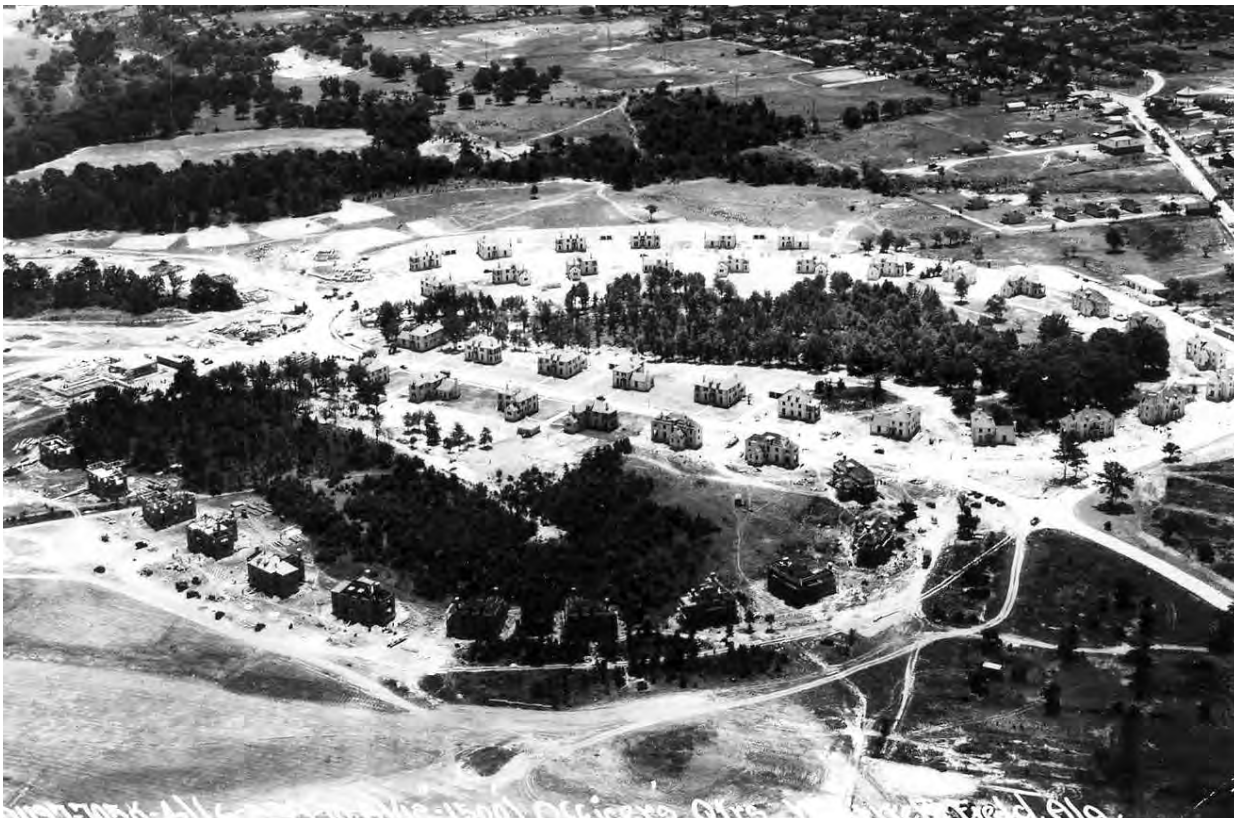
Aerial view of the new officer housing area under construction between 1932 and 1935. The officer houses exemplified the French Provincial architectural style to honor southern Alabama's colonial heritage as part of New France from 1702 to 1763.
