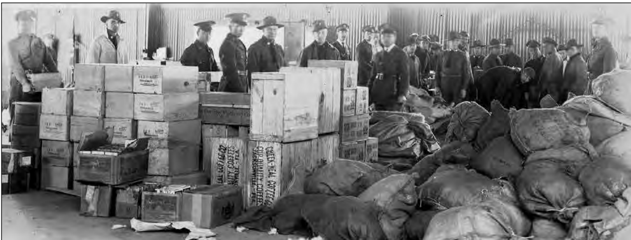
Flood relief stockpile in a warehouse on Maxwell Field
