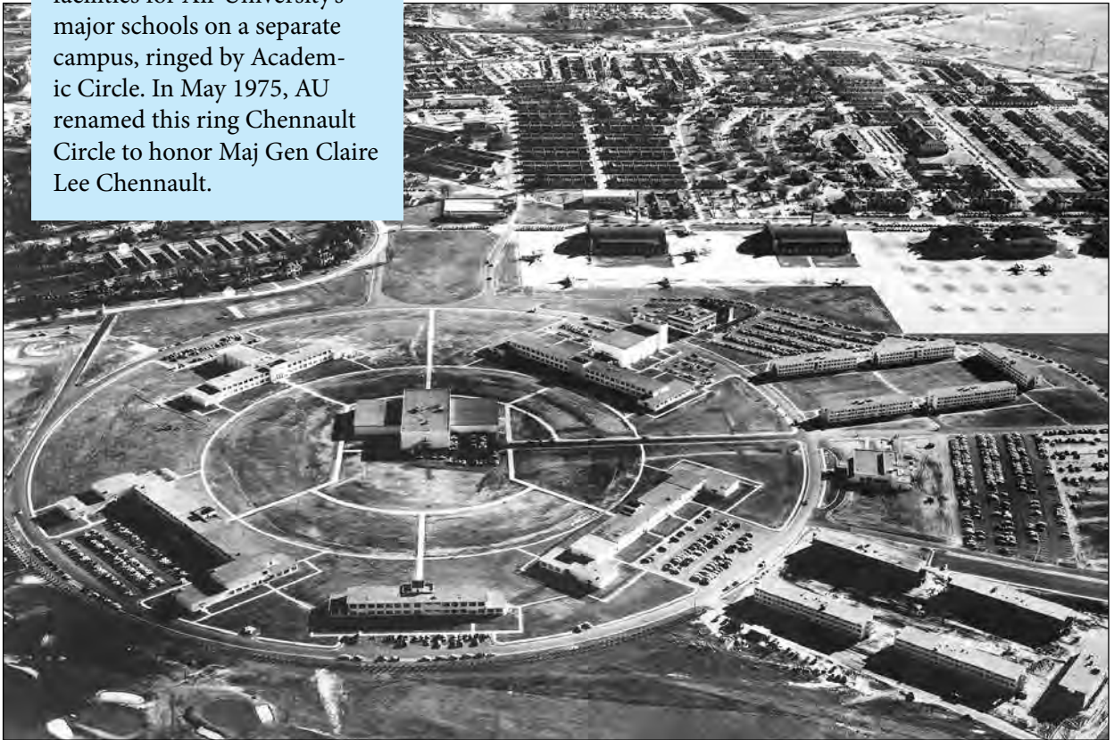
Aerial view of Academic Circle in 1958 after completion of the main schools along the circle and the Air University Library in the center and before landscaping
