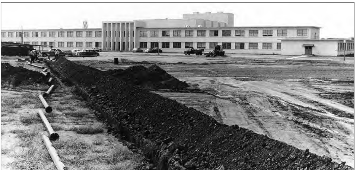
Underground utilities placement in front of the Air War College building
