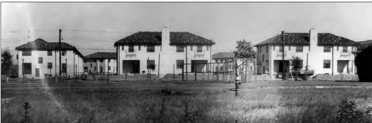
The two-story NCO duplexes after completion in September 1929. They still stand today on Mitchell Street.
