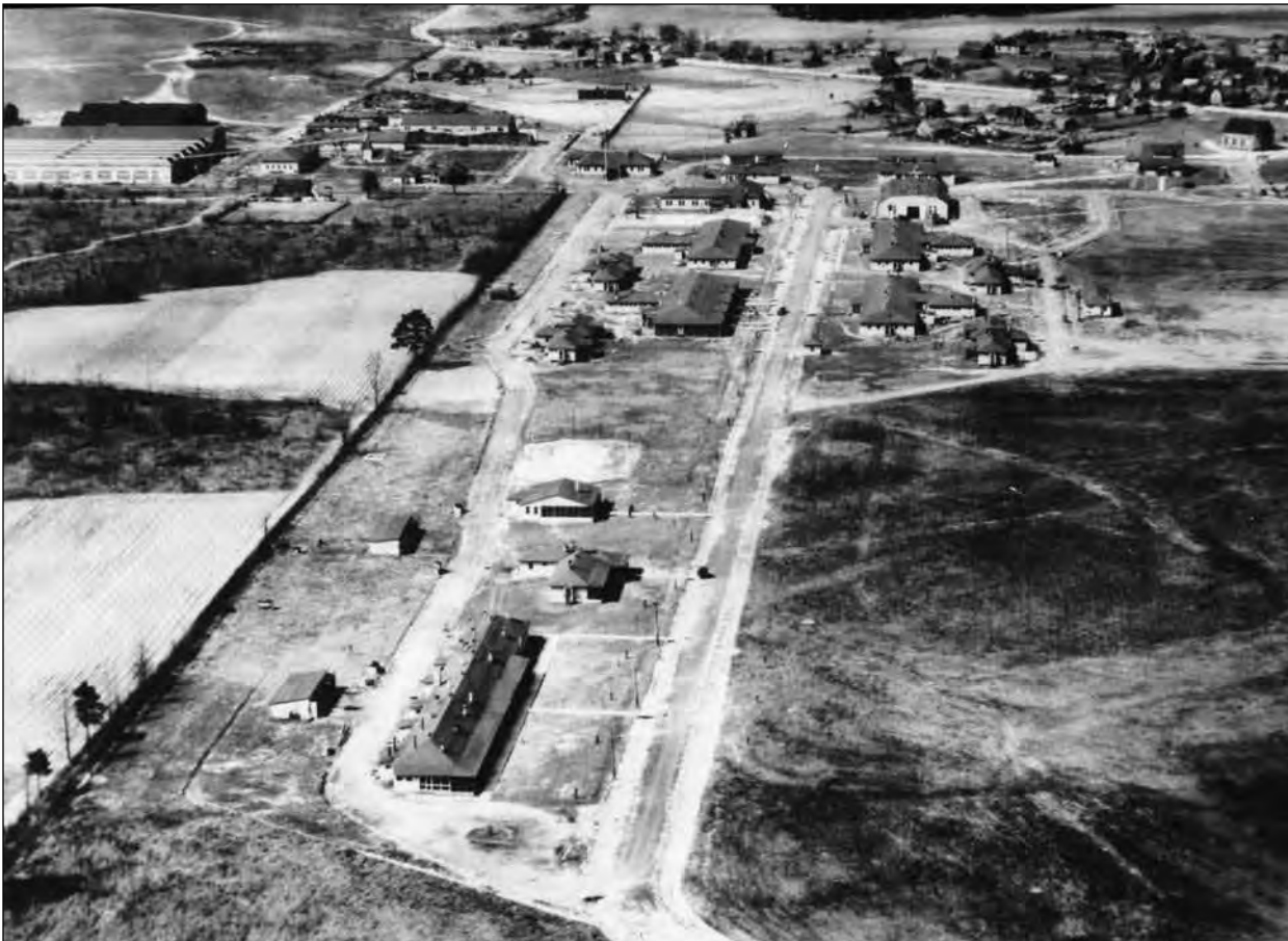
Aerial view of Aircraft and Engine Repair Depot no. 3 in about 1918. The depot's name changed to Aviation Repair Depot no. 3 soon after. Construction began on 8 April 1918 when the James Alexander Construction Company of Memphis, Tennessee, began erecting 52 wooden buildings on the site of the old Wright Field. The contractor completed the initial installation facilities, including three miles of Tarvia-surfaced roads, on 7 July 1918, just three months after construction began.
