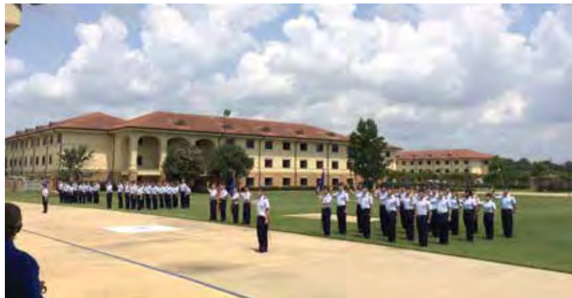
General Larry D. Welch Field, the OTS parade ground next to the OTS complex. The base constructed the parade ground from April through September 2006. The field was named in honor of retired Air Force general Larry D. Welch, commander of the Strategic Air Command, August 1985 to June 1986, and chief of staff of the Air Force, July 1986 to June 1990.
