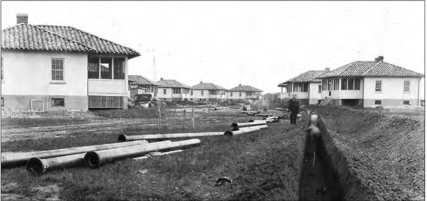
Some of the 13 permanent NCO housing structures on Maxwell Field as they neared completion in 1927
