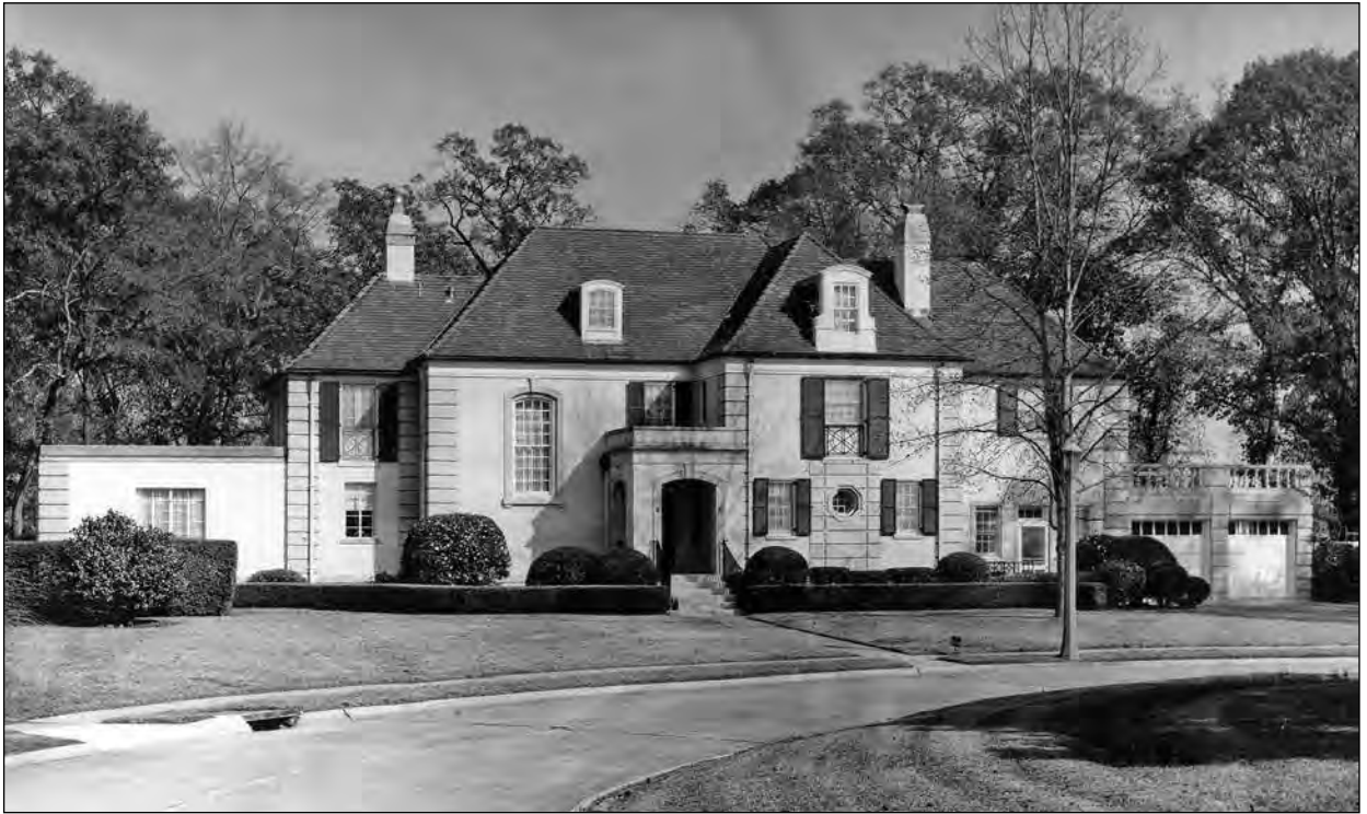
The post commander/ACTS commandant's quarters, seen here in the 1940s, is the largest within this housing area. It later became known as the Curry House after its first occupant, Maj John Curry. Since March 1946, it has served as the residence of the Air University commander.
