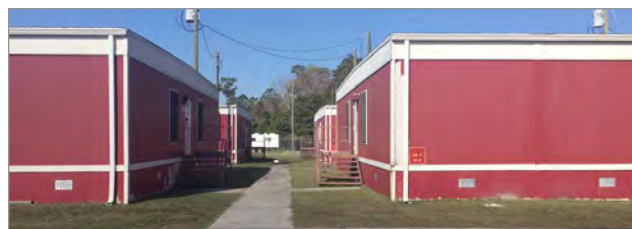
Relocatable Buildings at MCB Camp Lejeune
